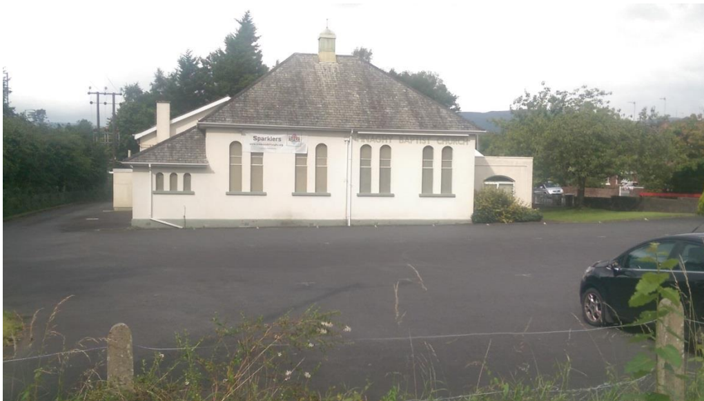
Photograph 6:3: Finaghy Baptist Church, Kingsway
