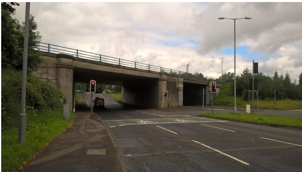
Photograph 6:1: M1 overpass at Black's Road
