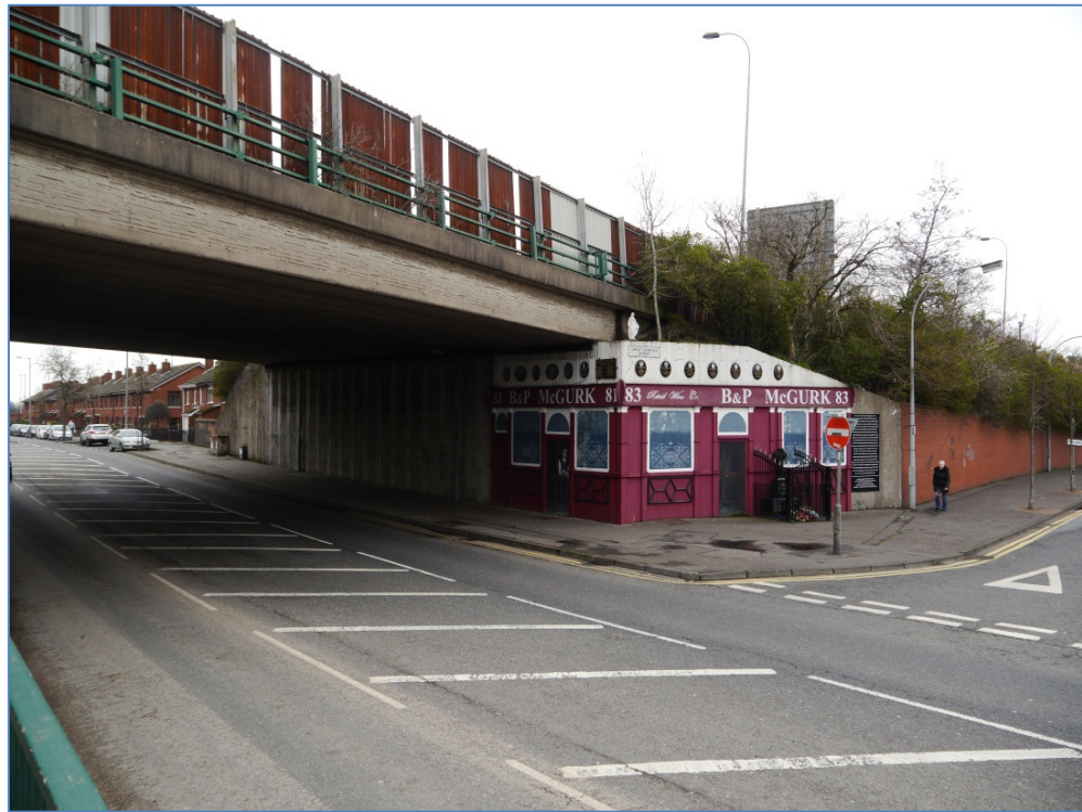
Figure 2.3.3 Southern elevation of North Queen Street Bridge
