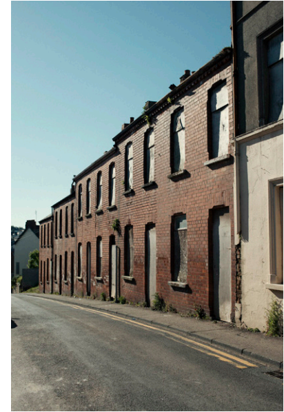
6 Existing derelict terrace houses at Kings Street.
