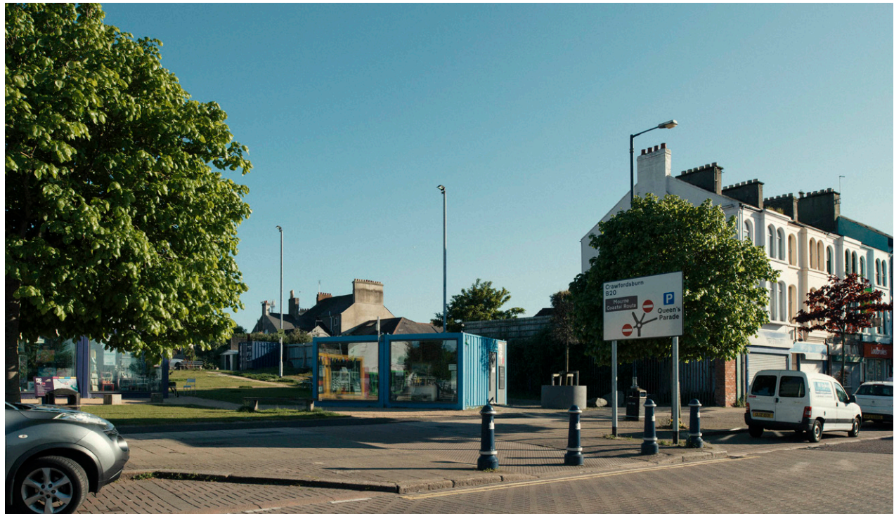
2 A view of the existing gap in the frontage along Queen's Parade.
