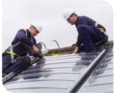
Installing solar thermal panels.
