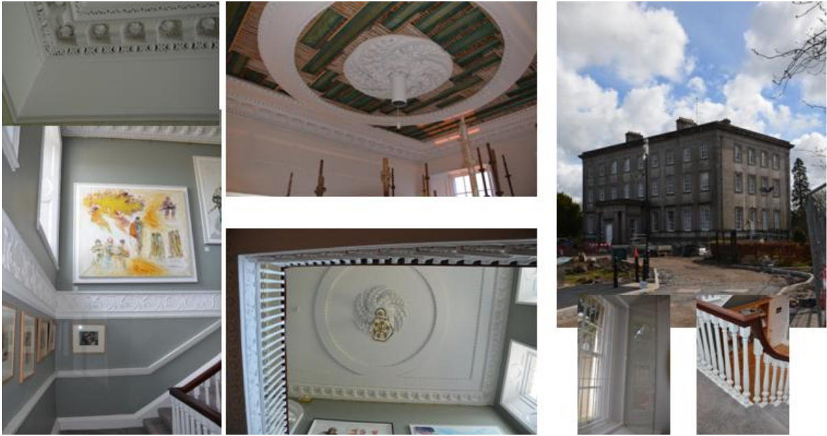
Bishop's Palace Armagh – repairs to interior plasterwork
