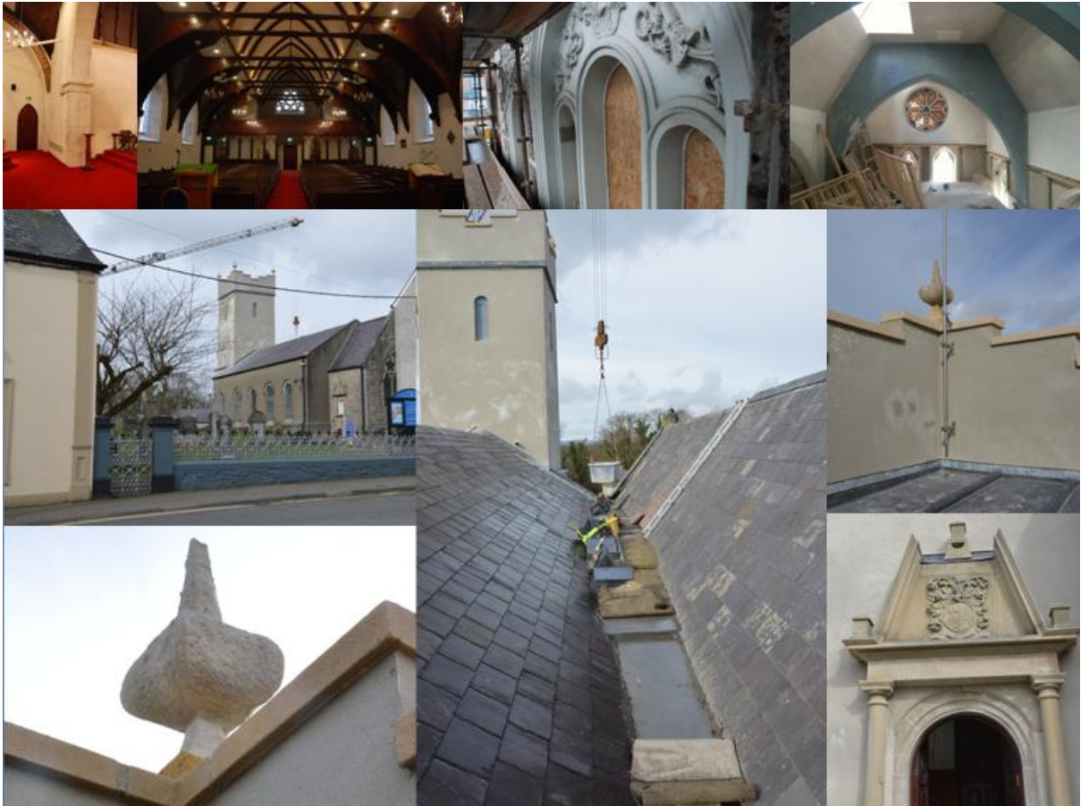
Derg Parish Church Castlederg – roof repairs
