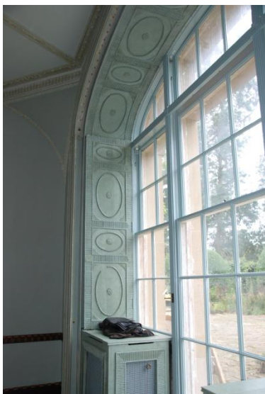
Repairs to window and linings Mount Stewart
