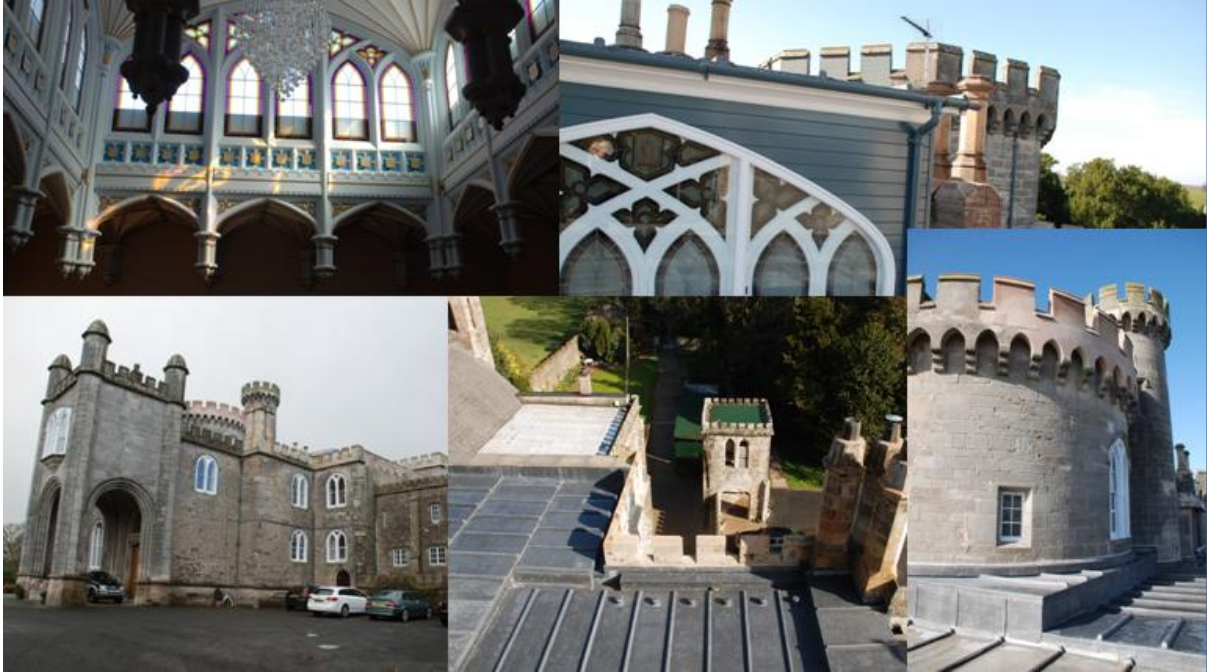
Killymoon Castle- roof repair works
