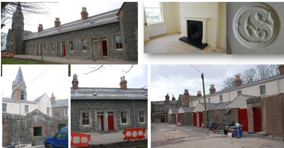
Conservation works at Charles Sheil's Housing, Killough
