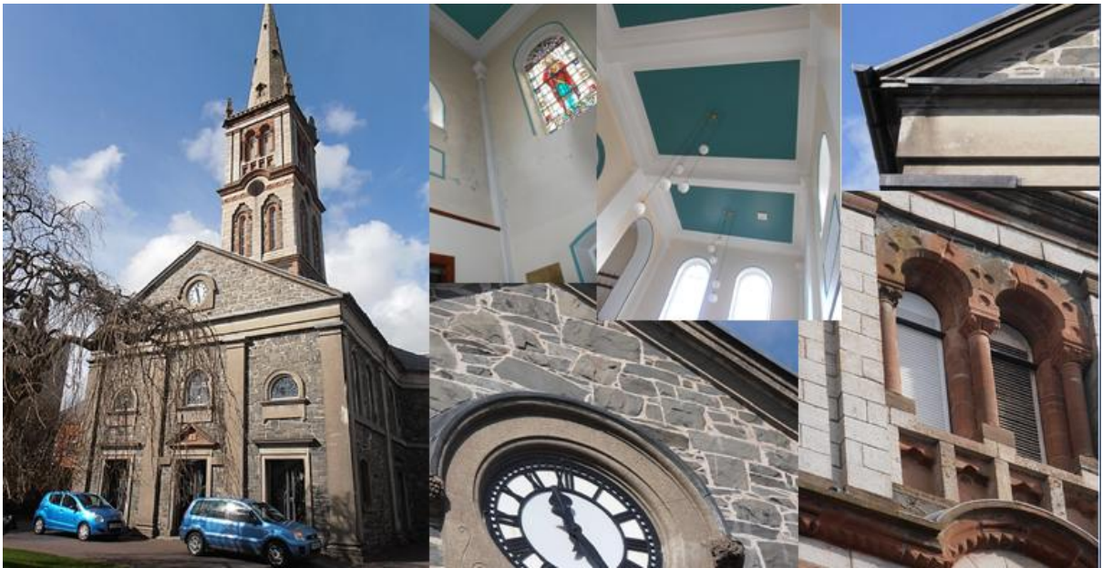
1 st Presbyterian Church Bangor – stone repairs
