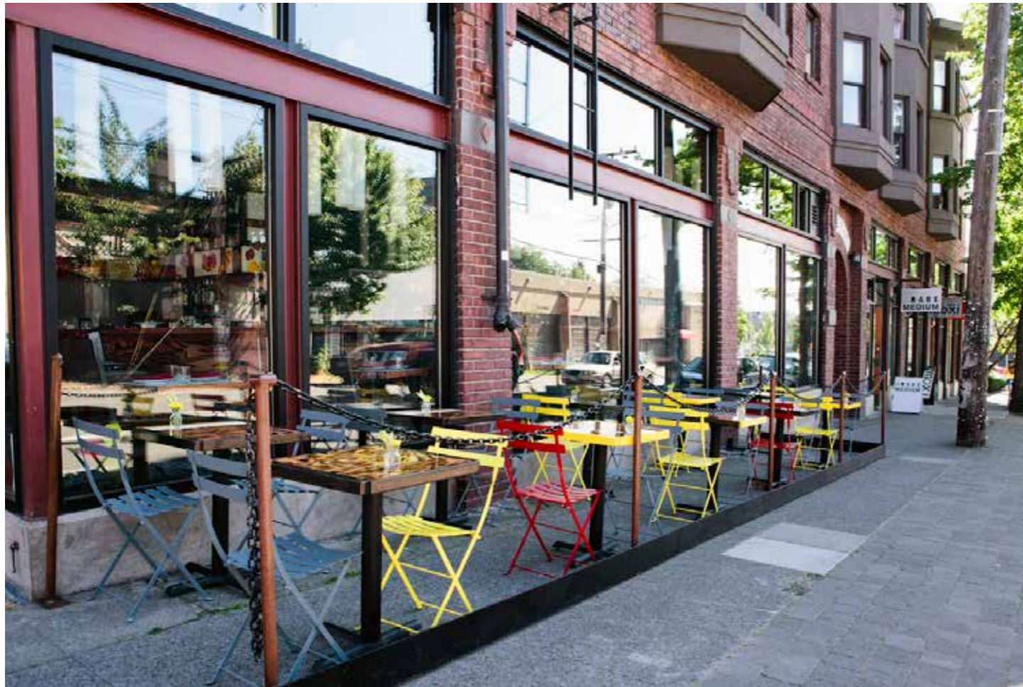
Example of Living Over The Shops (LOTS) and ground floor cafe culture
