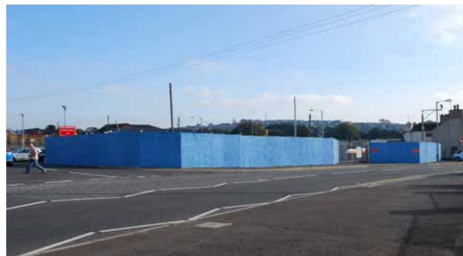
Construction of the new bus station
