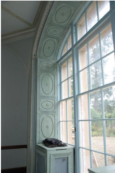
Repairs to window and linings Mount Stewart
