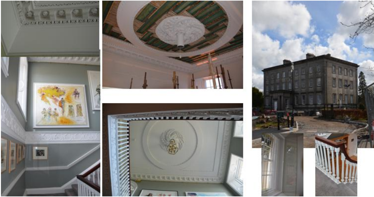
Bishop's Palace Armagh – repairs to interior plasterwork
