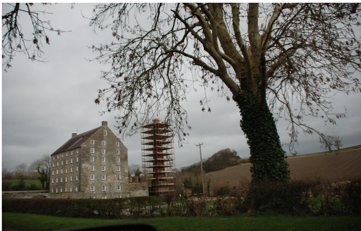
Ballydugan Mill and chimney
