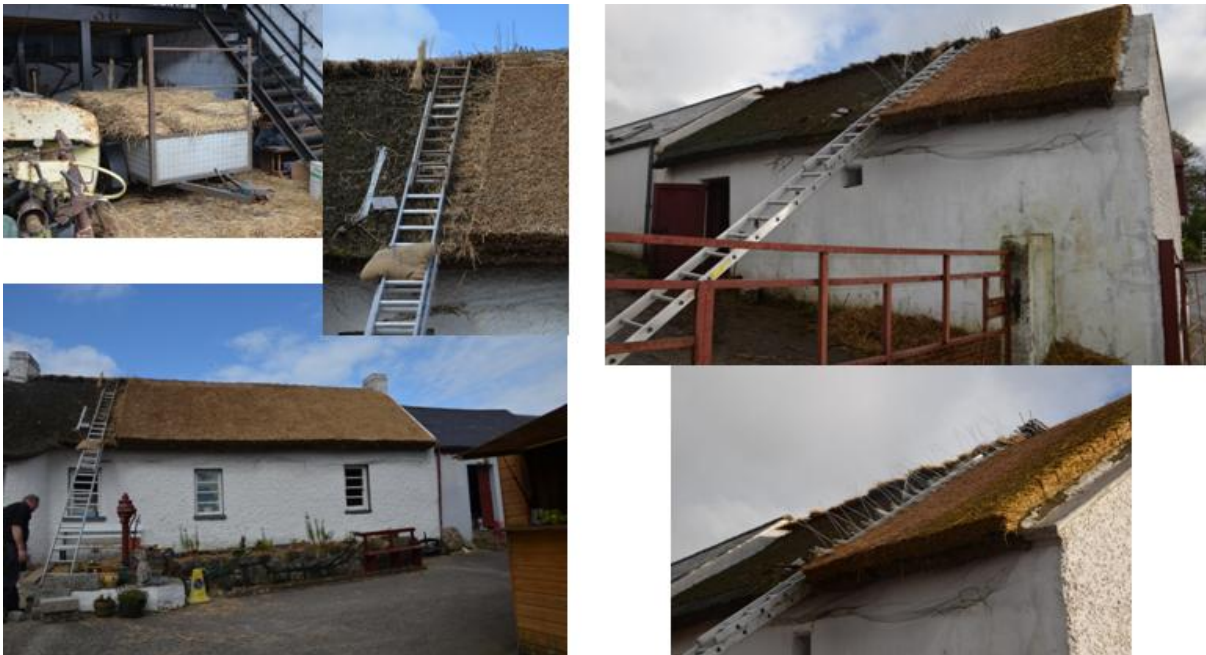
Thatching at Dan Winter's cottage
