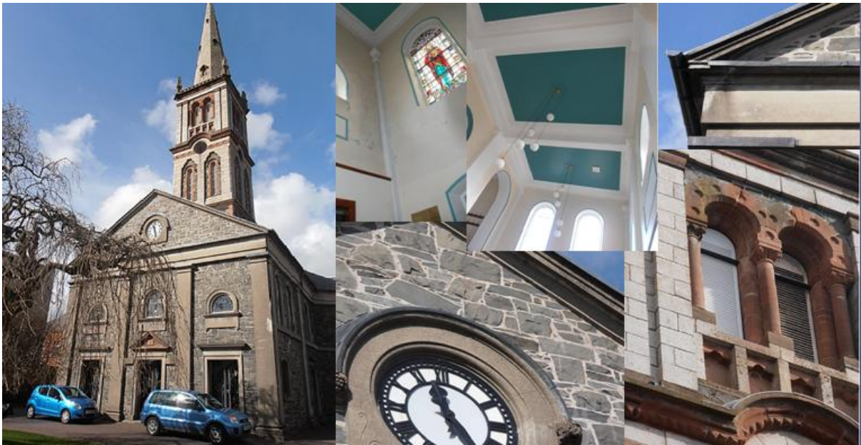
1 st Presbyterian Church Bangor – stone repairs
