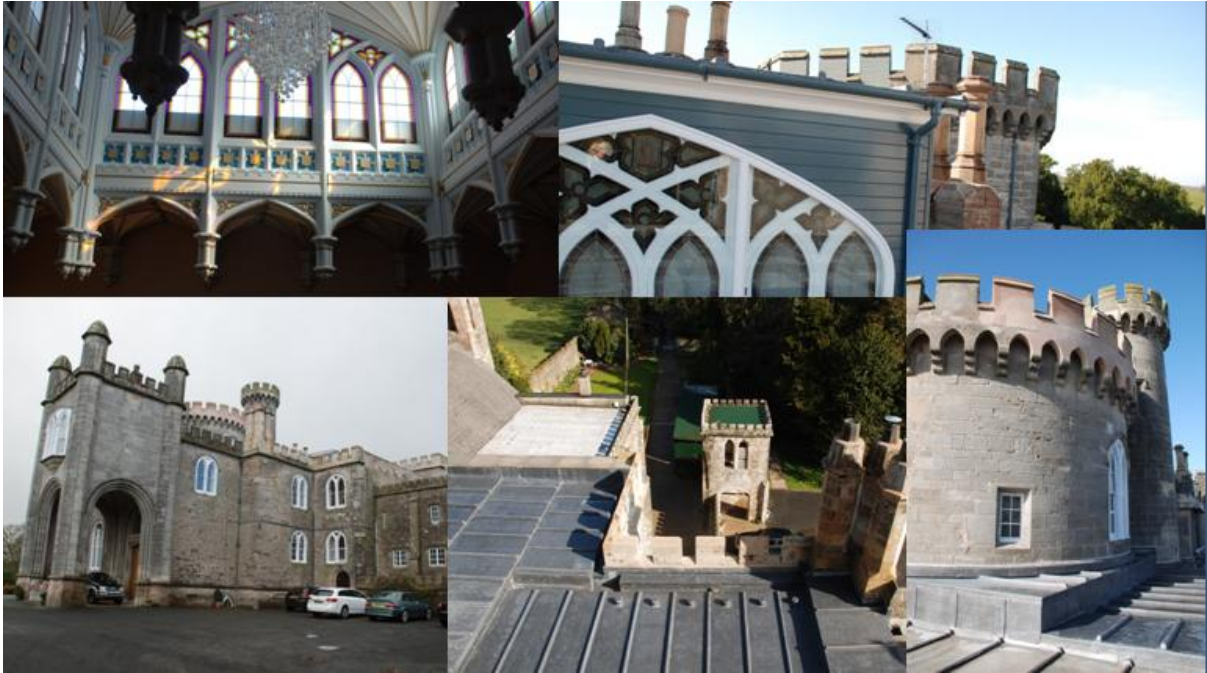
Killymoon Castle- roof repair works
