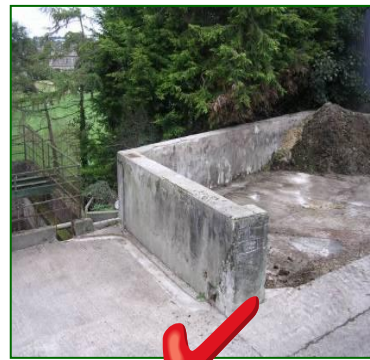
Photo 15 – Midden with all manure contained and run-off collected
