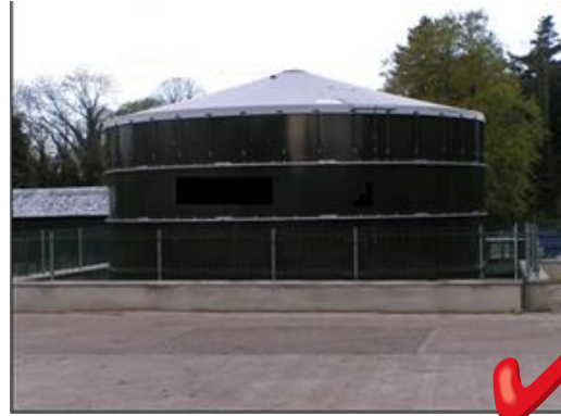
Photo 11 – Well maintained above ground slurry tank
