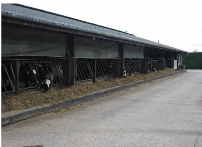
Photo 28 - Yard producing clean water.
