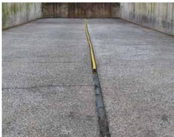
Photo 30 – Run-off from an empty and cleaned silo would be clean water.
