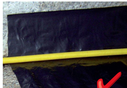
Photo 9 – Protecting silage pit wall-floor joints
