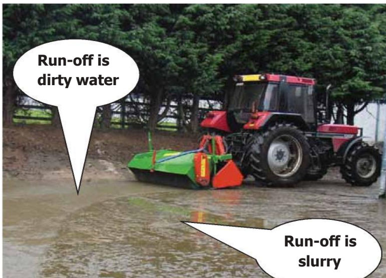
Photo 27 - The removal of slurry from yard areas will reduce the requirement to store slurry.
