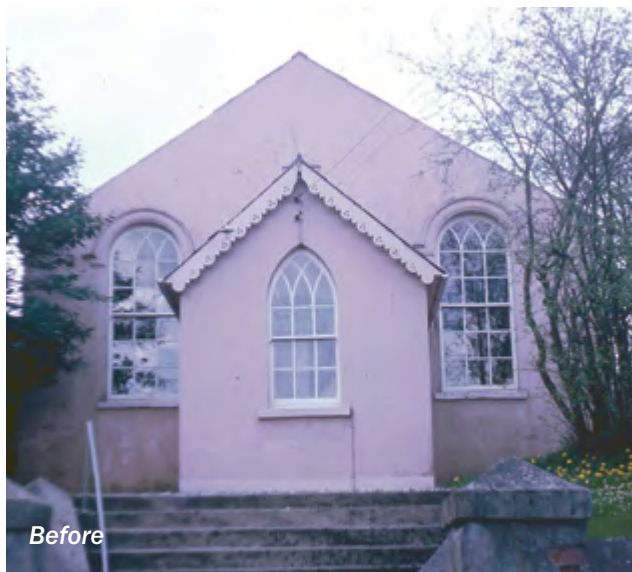
This listed chapel, built in 1818, was originally a building of significant local interest. Substantially rebuilt in 1982, it now has uPVC windows, fibre cement slates, pebble dash render and an entirely modern interior. The building no longer meets the test, and was delisted in 2010.
