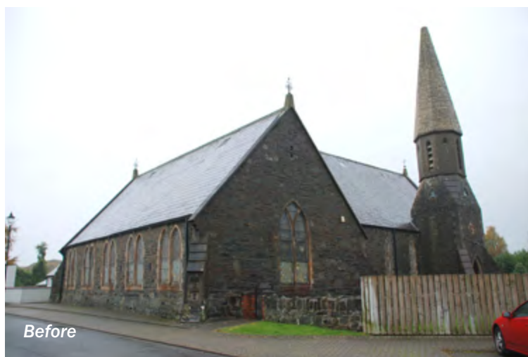
This listed chapel, built in 1818, was originally a building of significant local interest. Substantially rebuilt in 1982, it now has uPVC windows, fibre cement slates, pebble dash render and an entirely modern interior. The building no longer meets the test, and was delisted in 2010.
