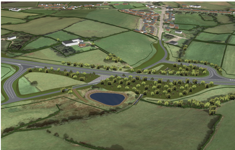
Indicative Compact Grade-Separated Junction
