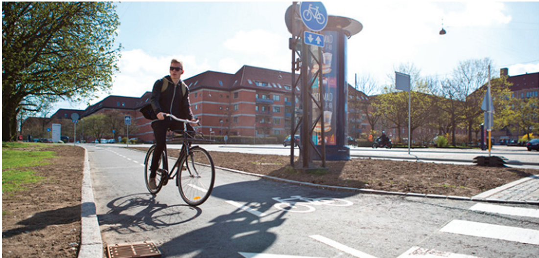
Figure 15: Two-way bicycle track along Hans Knudsens Plads
