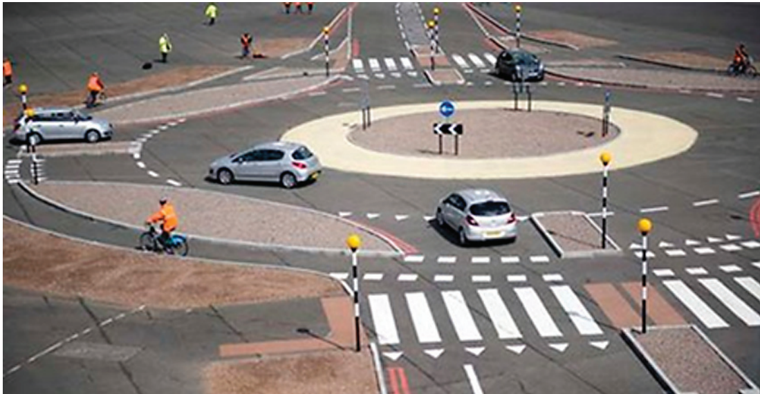
Figure 4: A typical Dutch roundabout
