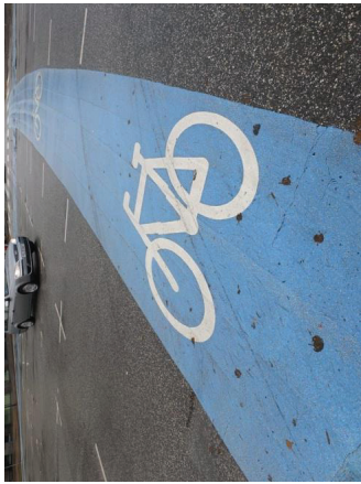
Cycle lane demarked at road junction - Copenhagen
