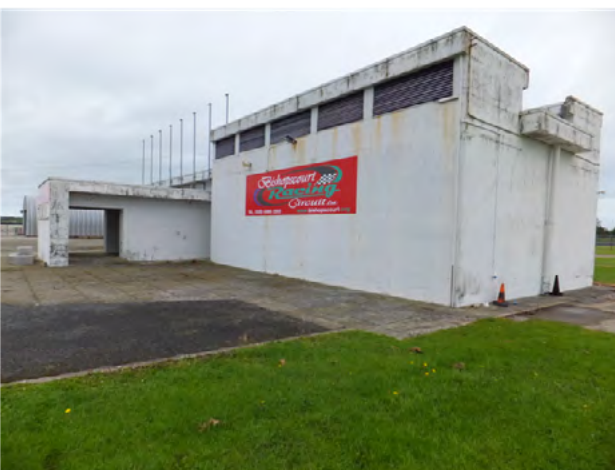
Figure 25. The control and reporting post at Bishops Court (DHR 00032:048)
