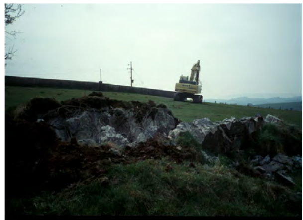
Figure 34. Demolition of a pillbox (DHR 00080:032) outside St Angelo airfield, Co. Fermanagh, 2004
