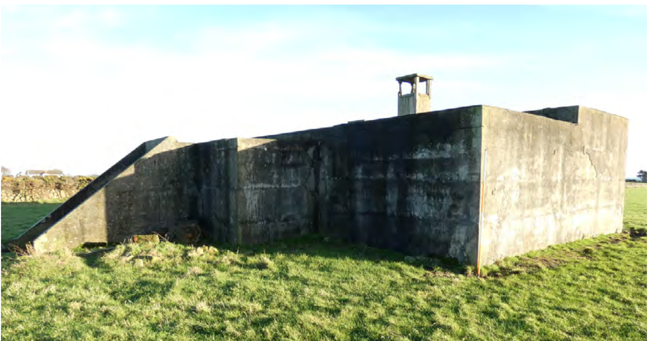
Figure 16. Transmitter block (DHR 00167:006) at Kilkeel Chain Home radar station, Co. Down
