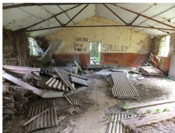
Figure 29. Asbestos sheeting stored at the flight offices and crew room, Limavady, Co. Londonderry (DHR 00070:063)
