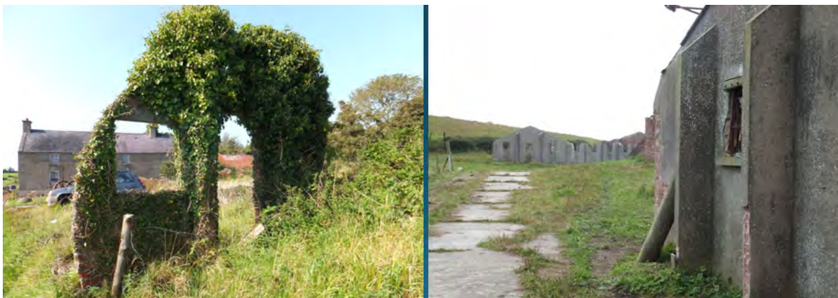
Figure 9. Barracks at Ballyhalbert, Co. Down (DHR 00028:060); picket hut and ablutions block at Kirkistown, Co. Down (DHR 00040:040, 044)
