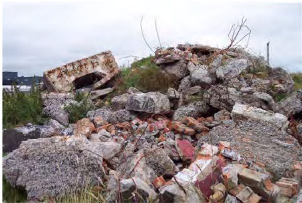
Figure 33. Demolition of a strongpoint (DHR 00087:013) at Newtownards prior to development in 2004
