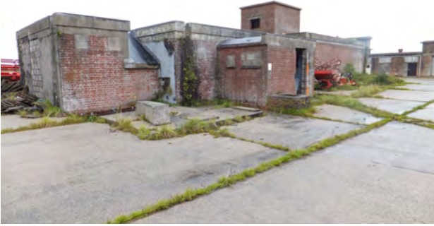
Figure 24. The radar modulator building at Bishops Court, Co. Down (DHR 00032:210)
