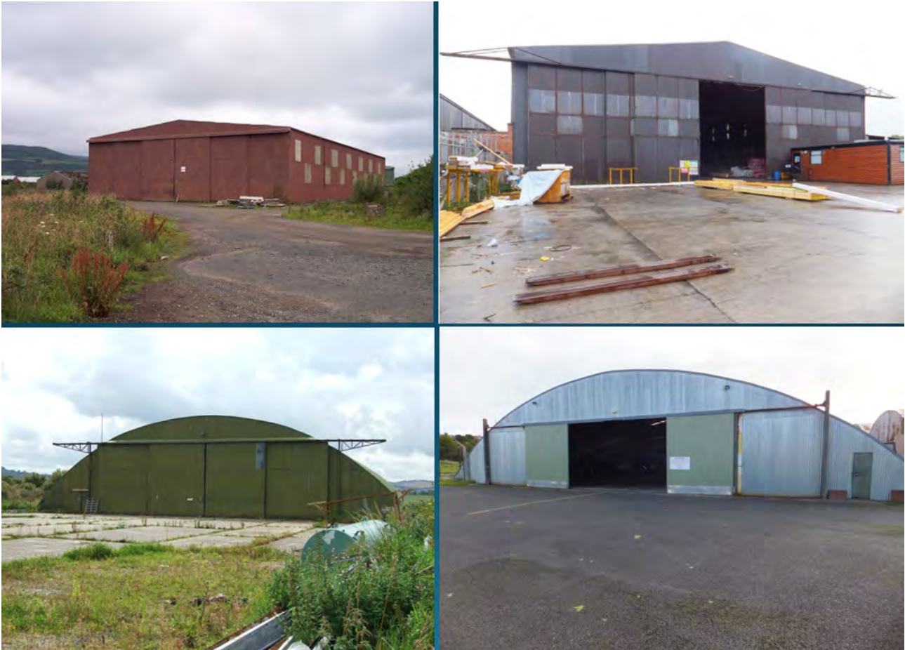
Figure 7. A Bellman hangar at Limavady, Co. Londonderry (DHR 00070:034); A T2 hangar at Maghaberry, Co. Antrim (DHR 00072:014); Fromson Hangar at Eglinton, Co. Londonderry (DHR 00037:017); Blister Hangar at Newtownards, Co. Down (DHR 00087:006).
