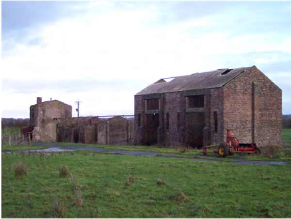
Figure 8. A Bombing Teacher, Link Trainer and Turret instructional building at Mullaghmore, Co. Londonderry (DHR 00075:36, 37, 38)
