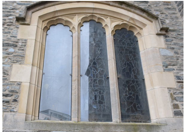
Deeply in set the protective Glazing – St Columb's cathedral Derry/Londonderry
