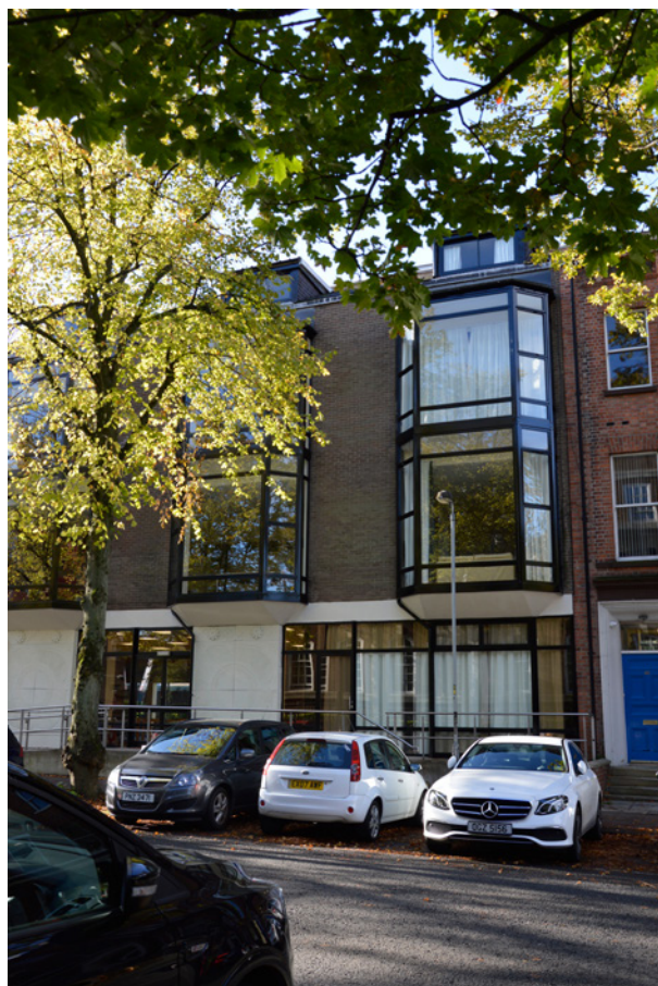
Curtain walling at Catholic Chaplaincy, QUB
