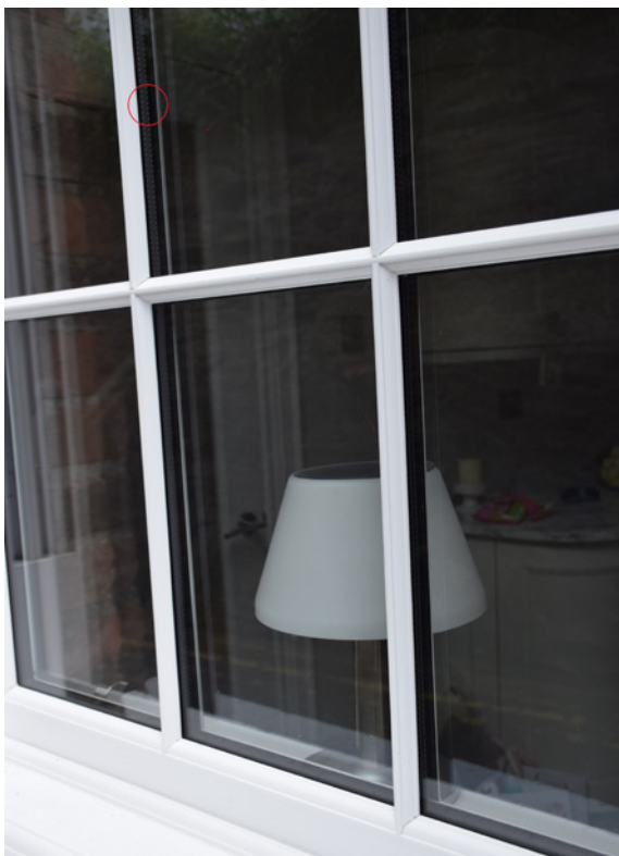
The wide edge seal is visible.
