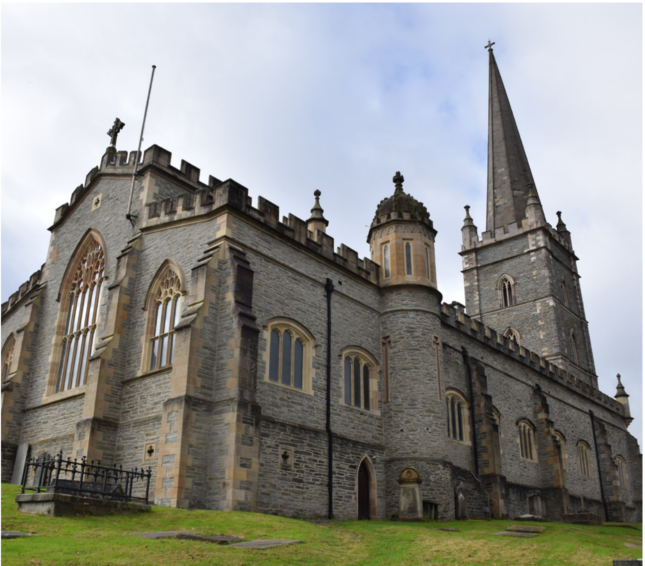
St Columb's cathedral Derry/Londonderry - The protective glazing is inset deeply; this results in considerably less impact on the overall aesthetic of the building.
