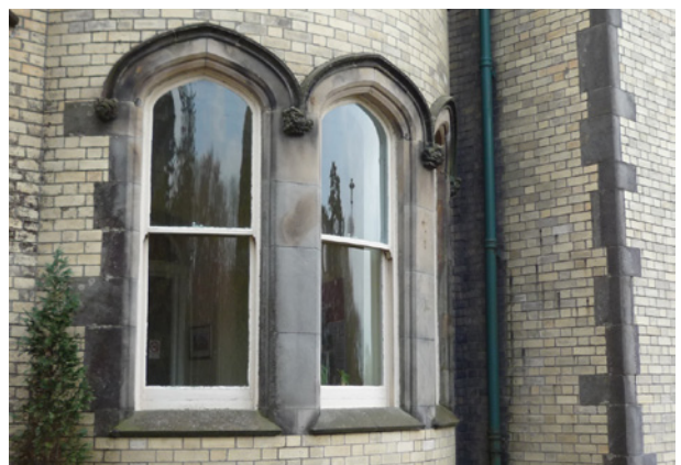
Curved sash windows with no glazing bars- note horns strengthening the mid rail.
