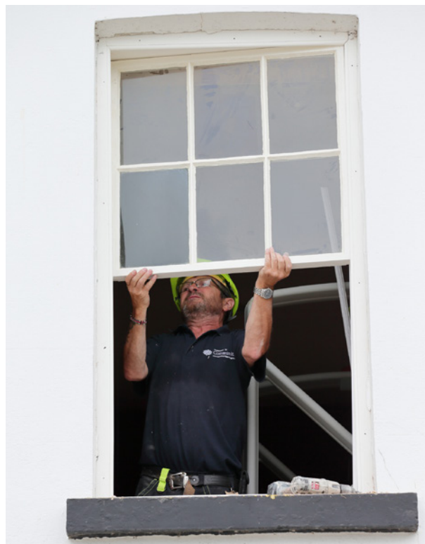
Replacement of historic windows
