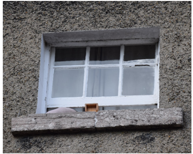
Early sash window, Armagh – sash moves vertically into a pocket.
