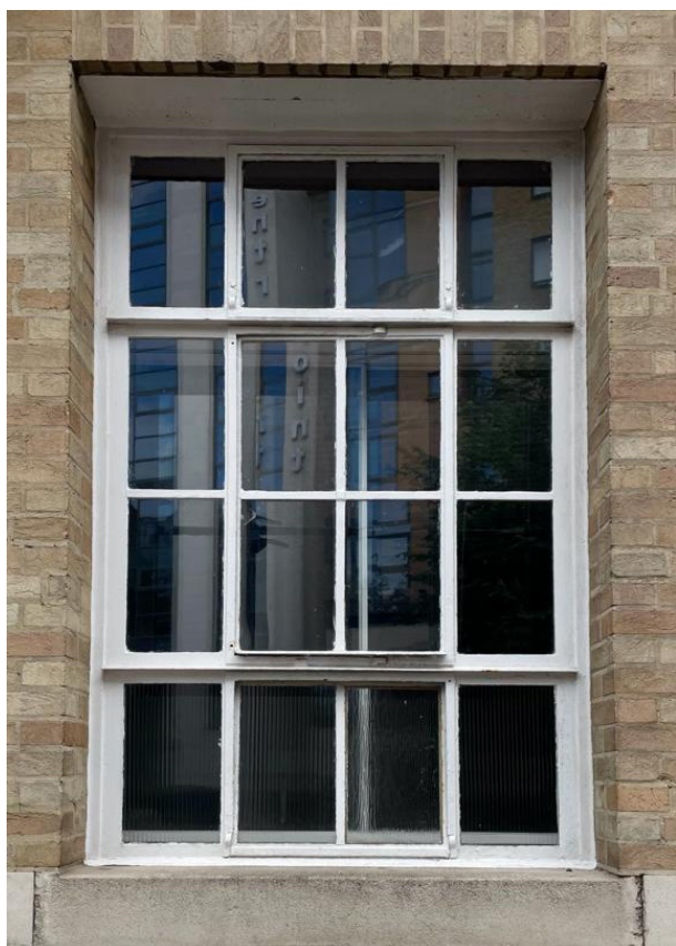
Crittall Window at BBC broadcasting House, Belfast
