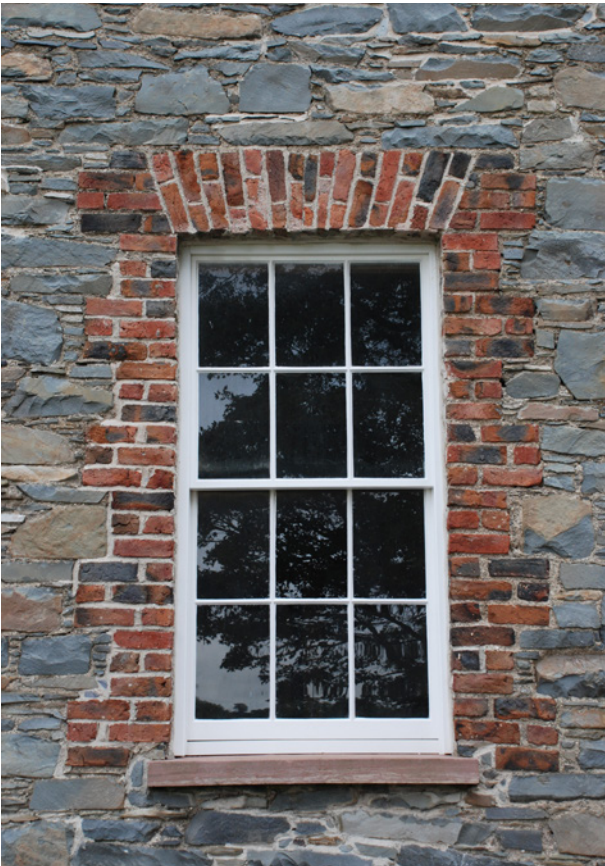
Typical Double Hung Sash Window
