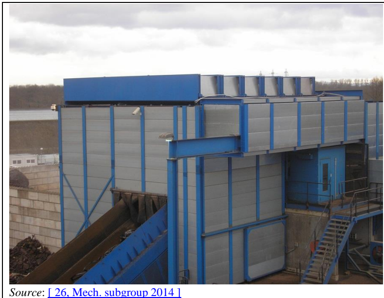
Figure 3.24: Splitter silencers at the roof of a shredding plant
