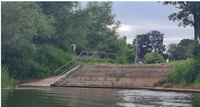
Concrete canoe steps and slipway, river Suir Clonmel
