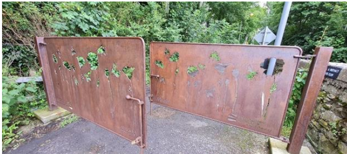
Street Furniture Local branded gate. Suir Blueway Clonmel, Corton steel
