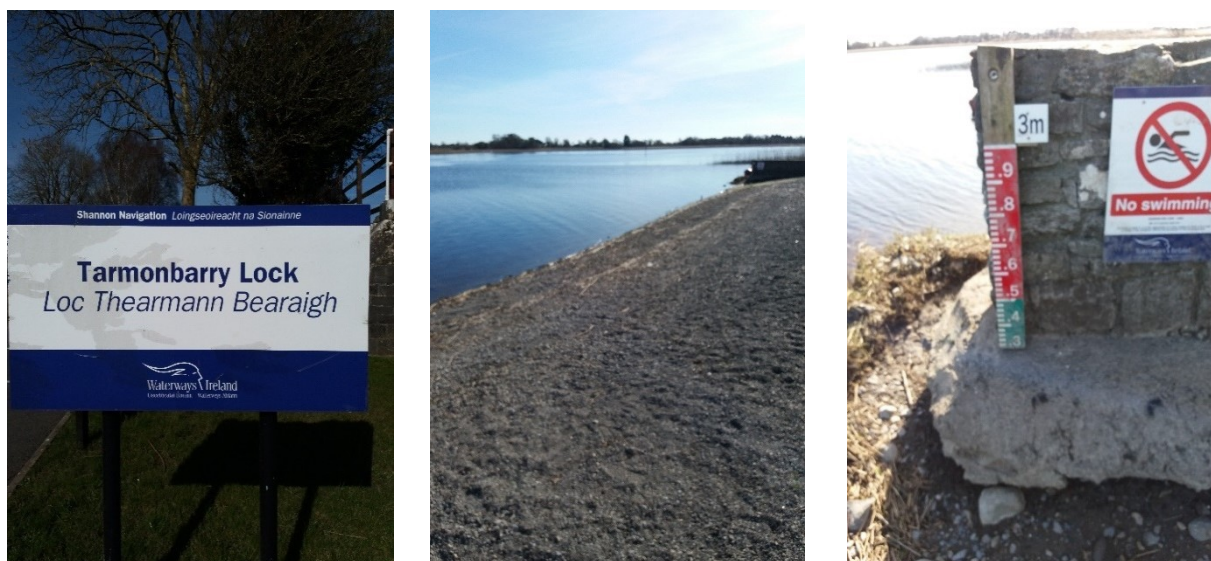
Figure 13: Slipway and Water Gauge at Tarmonbarry Lock
