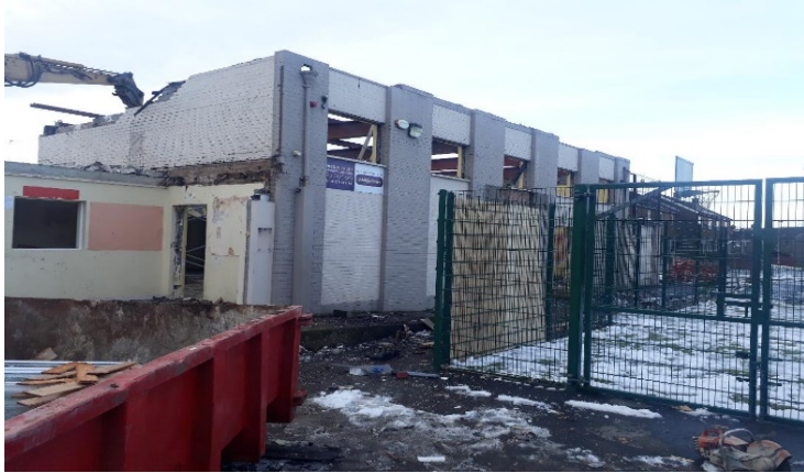
Building while under construction
