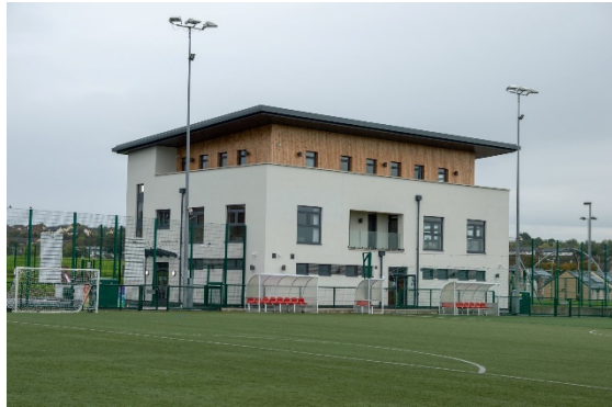
Leafair Pavilion Construction
