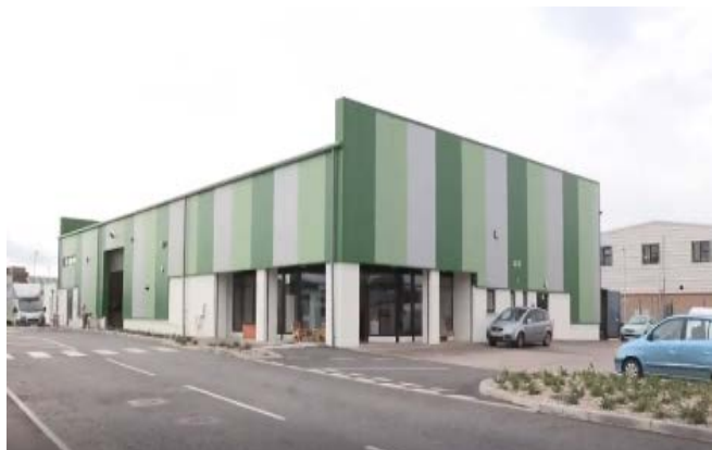
4Rs Recycling Facility at Pennyburn
