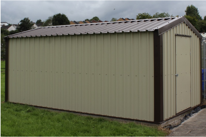
New storage shed - Derrybeg
