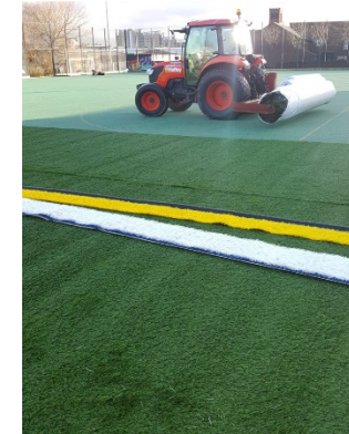
Laying of 3G pitch at Blythfield
