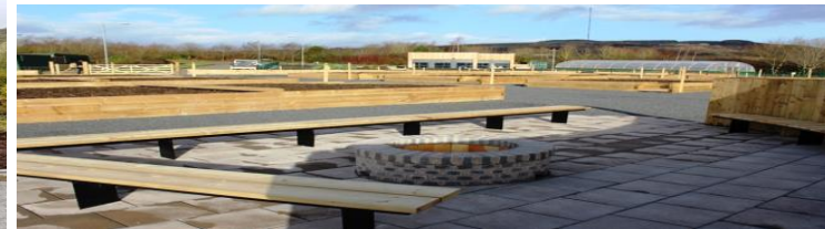
Completion of the development
