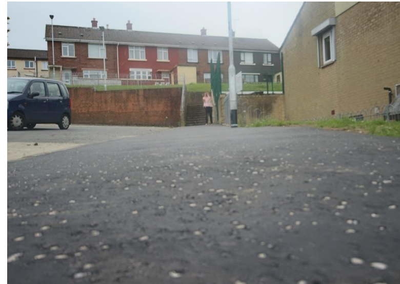
Resurfacing works have completed at Derryview
