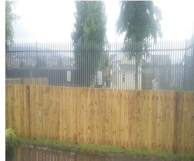
New fencing in place
