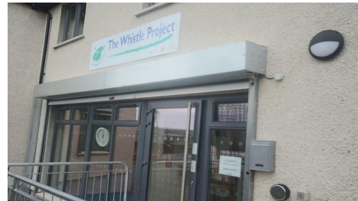
Renovation complete and ready for use
