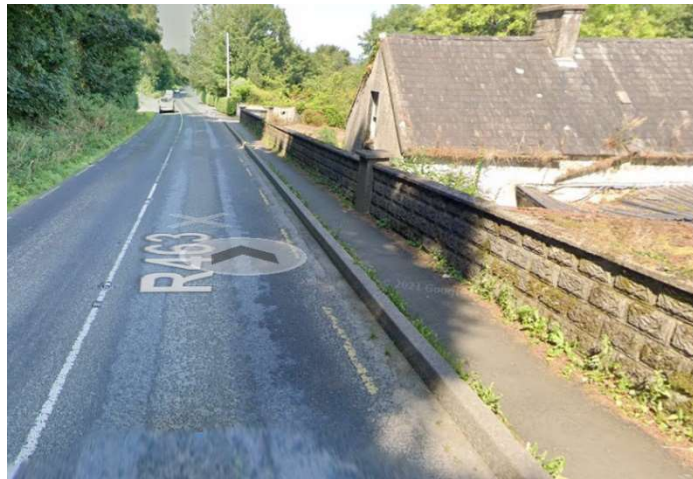
Figure 10: Property Adjacent R463 in in Ballyvalley
