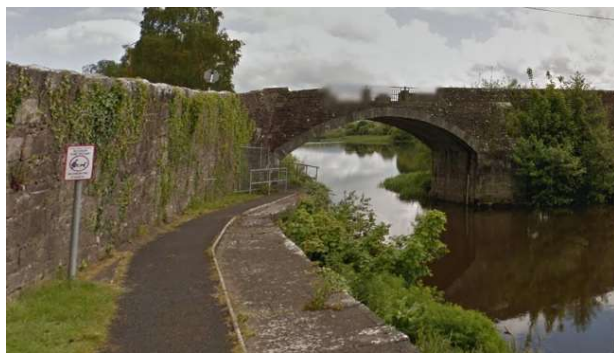
Figure 12: Existing Path Under O'Brien's Bridge
