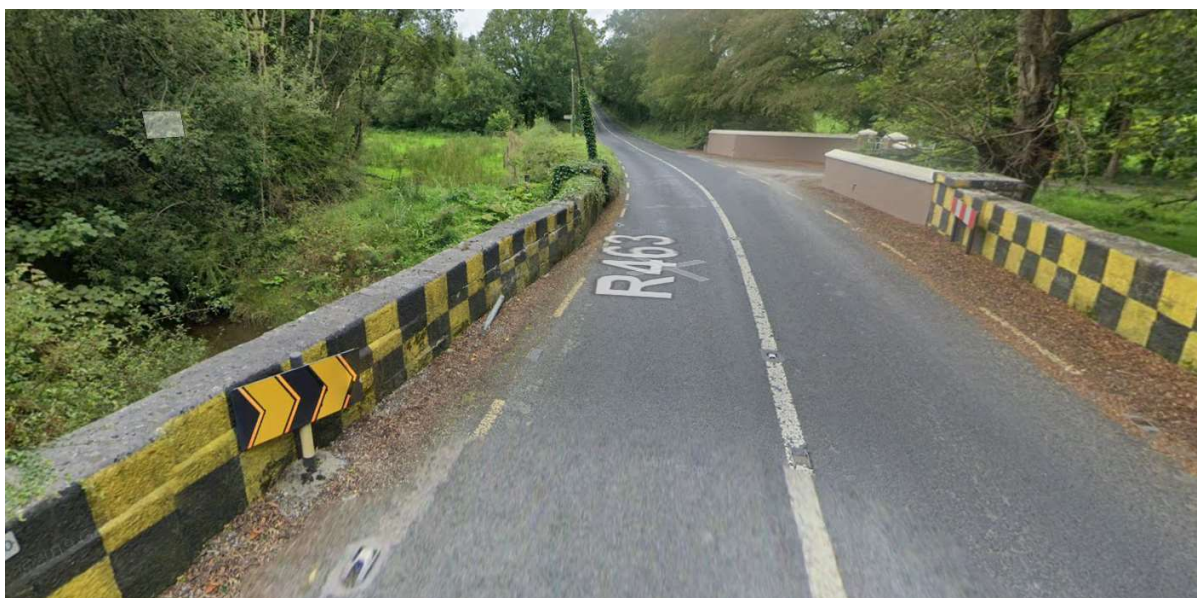
Figure 24: R463 Crossing of the Ardclony River
