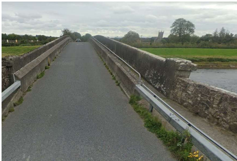
Figure 18: Existing Bridge over Shannon Head Race in Cloonlara
