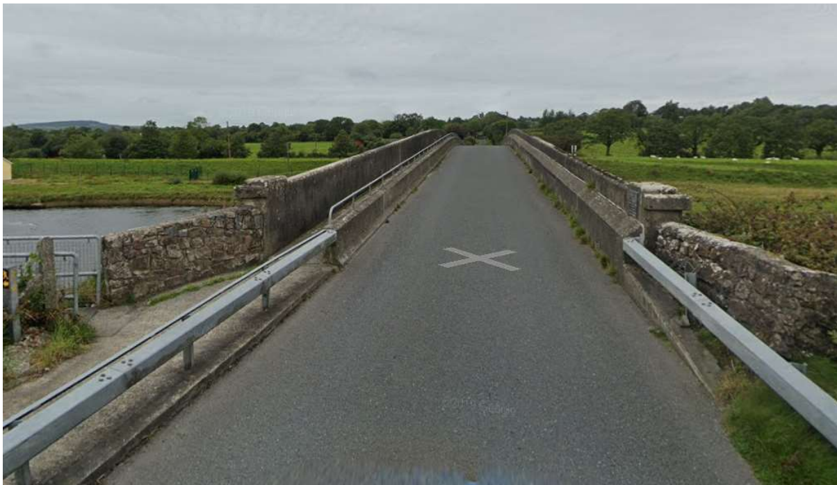
Figure 25: Existing Bridge over Shannon Head Race in Cloonlara
