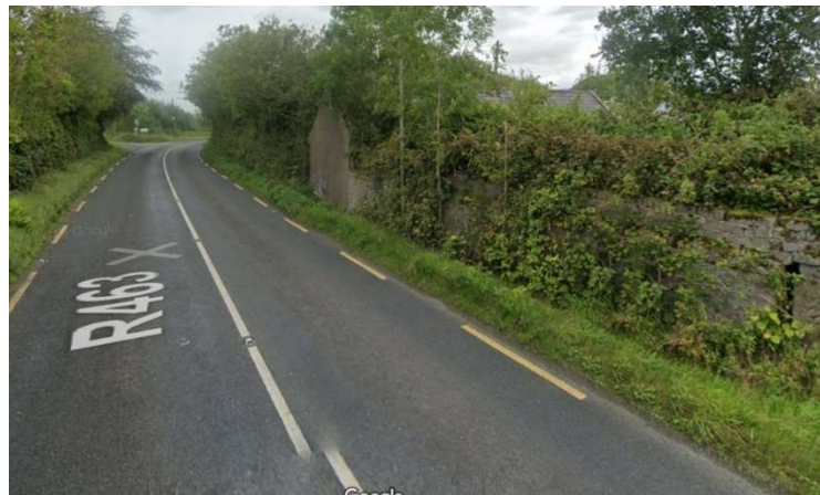
Figure 13: Shed and Wall along R463 in Cloonfadda
