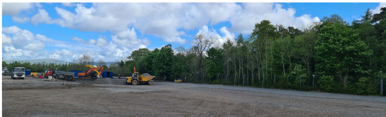
Site groundworks for the Newforge Shared Space.
