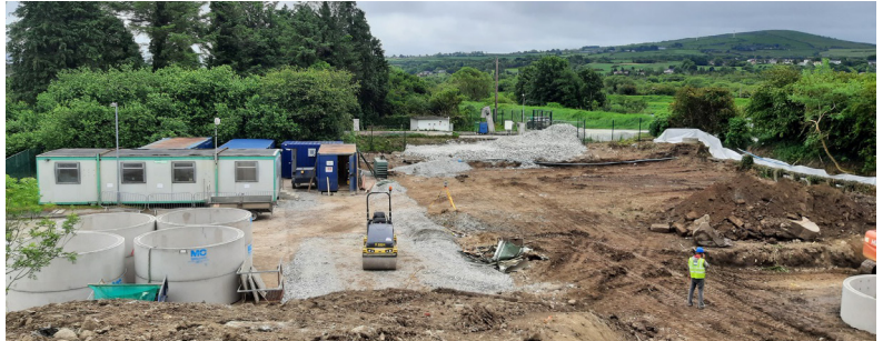
Early construction works at the Lifford site.
