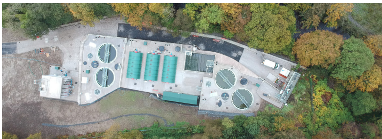
Aerial shot of the SWELL upgrade at the Donemana site.
