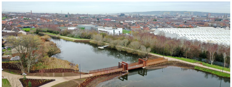
An aerial photo of the work completed to date at Springfield Dam.
