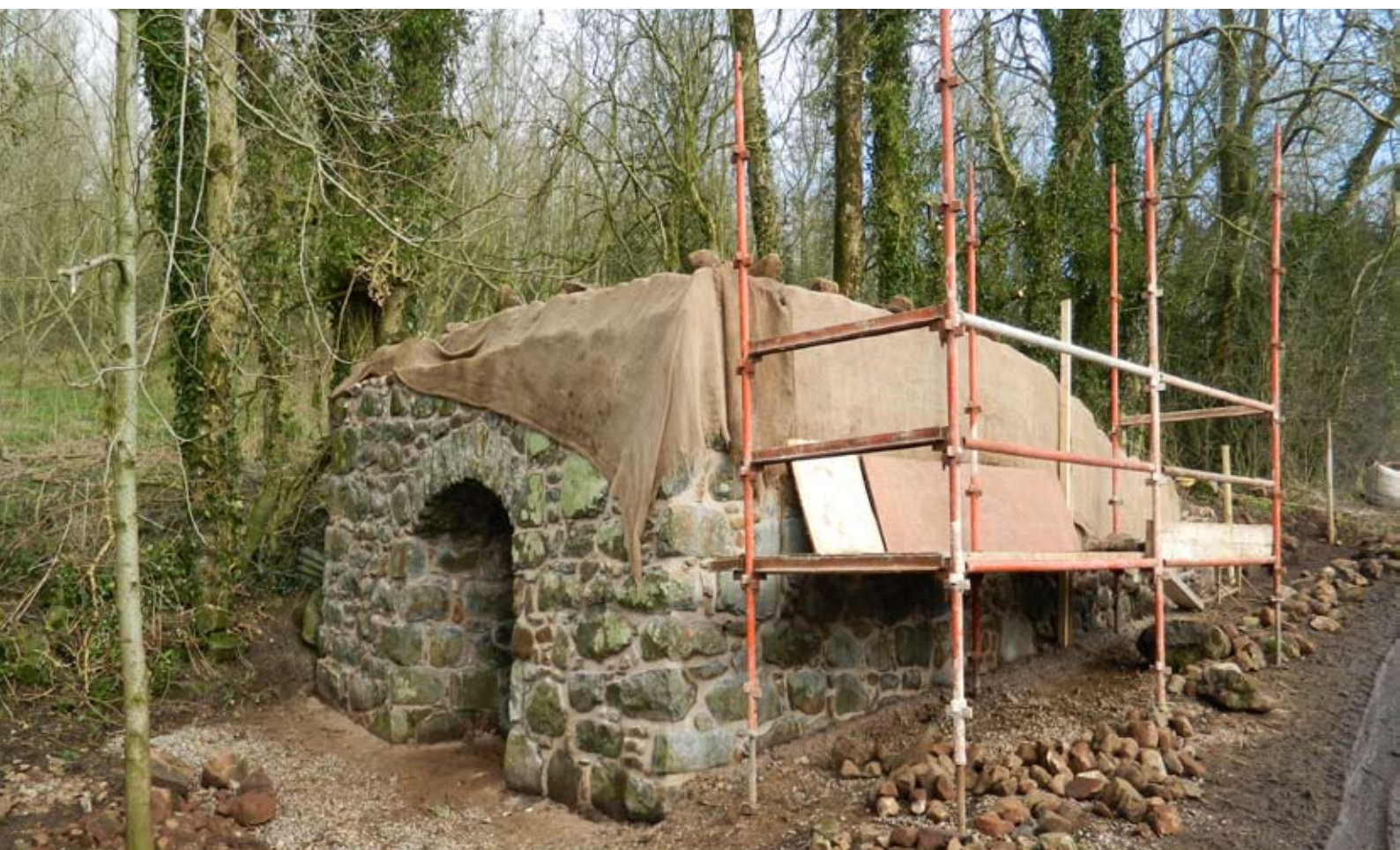
Lime kiln restoration at Gortakilly, Co. Londonderry © Sperrins Gateway Landscape Partnership
