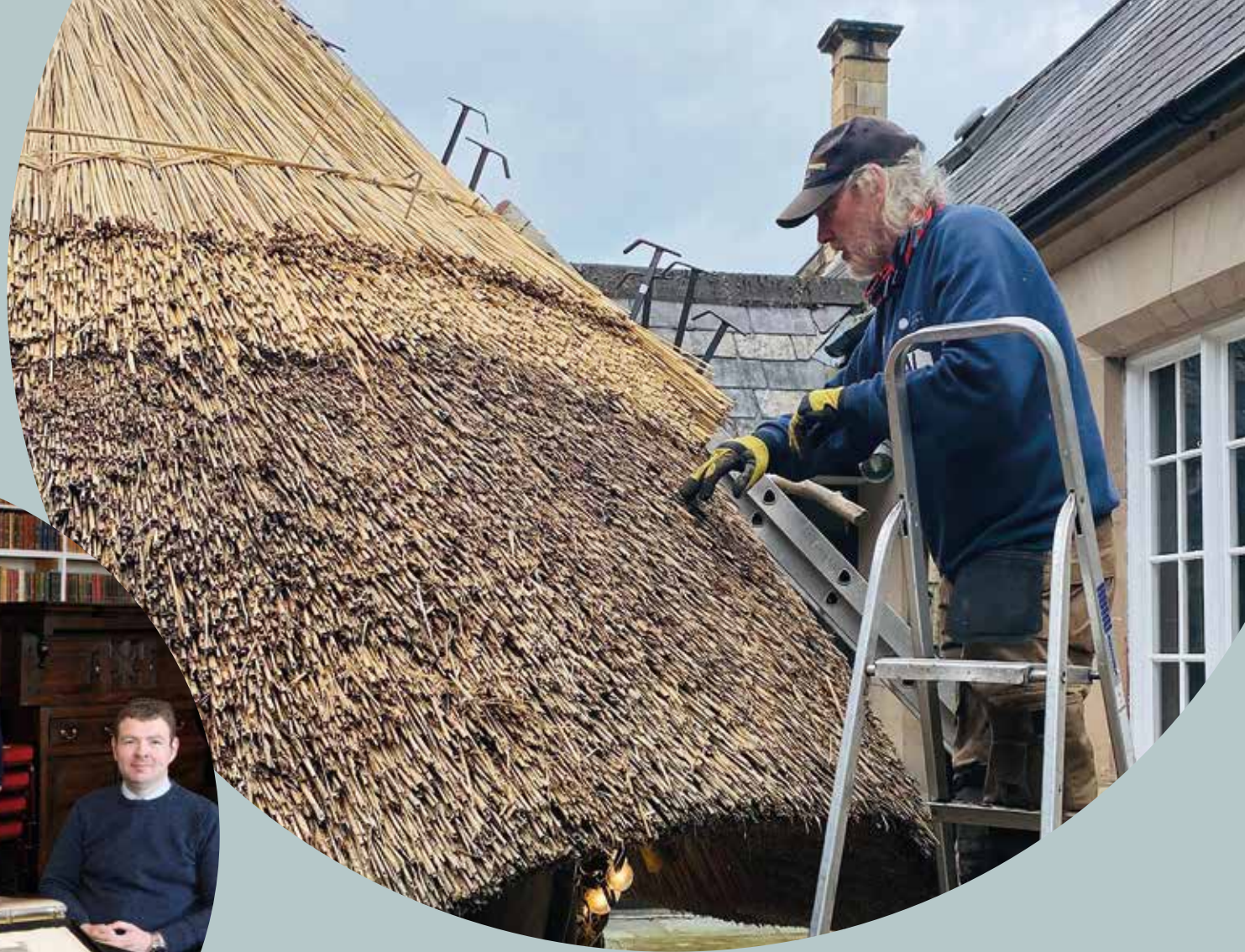
Rethatching of the monks cell at North Down Museum. Photograph courtesy of North Down Museum.
