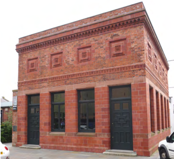
Belfast Gasworks Meter House
