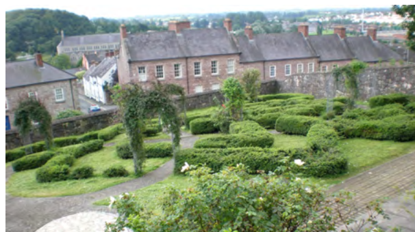
Roofs stepping downhill in Armagh
