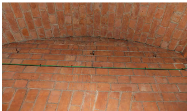
Brick barrel vault supported floor above,
