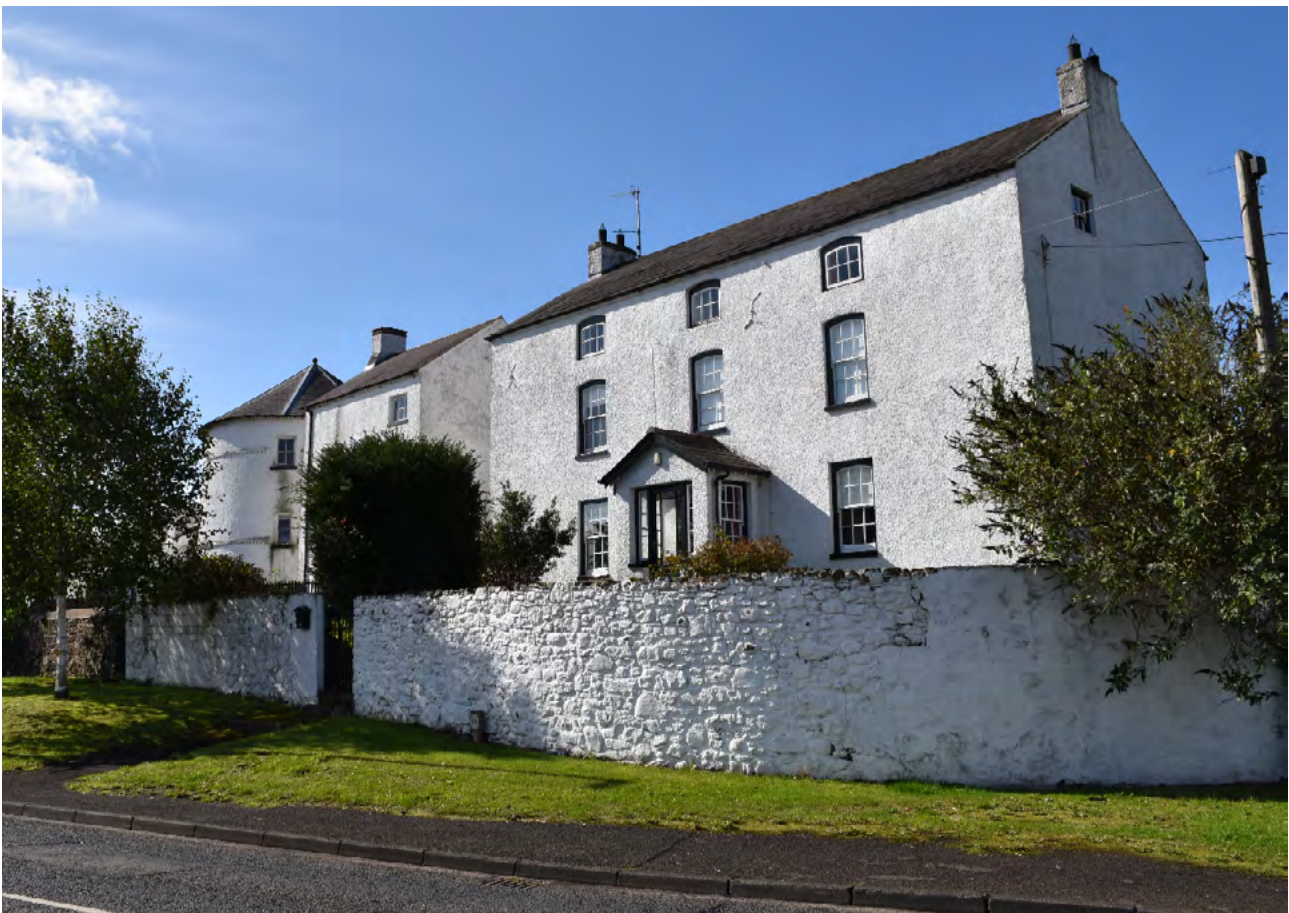
Bellaghy Castle, limewashed rubblestone walls
