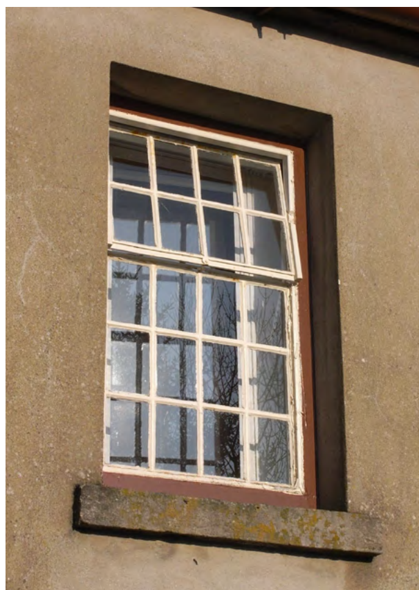
Metal window with pivot turn opener
