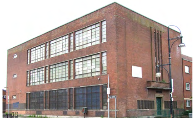
20th century steel windows
