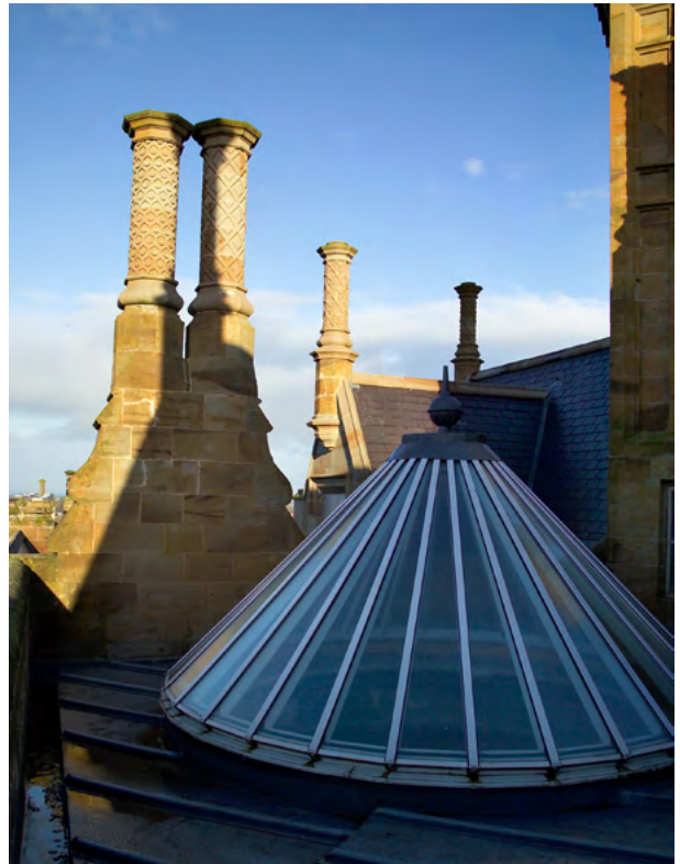
Complex roof with glass, lead and slated elements
