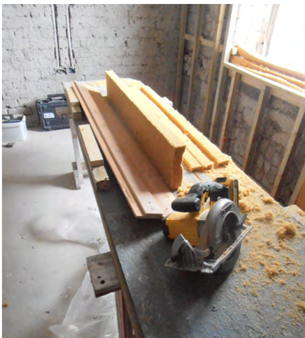
Wood fibre insulation on site
