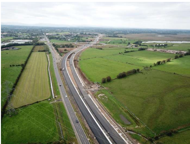
Arial view looking west – Toome Bypass tie-in
