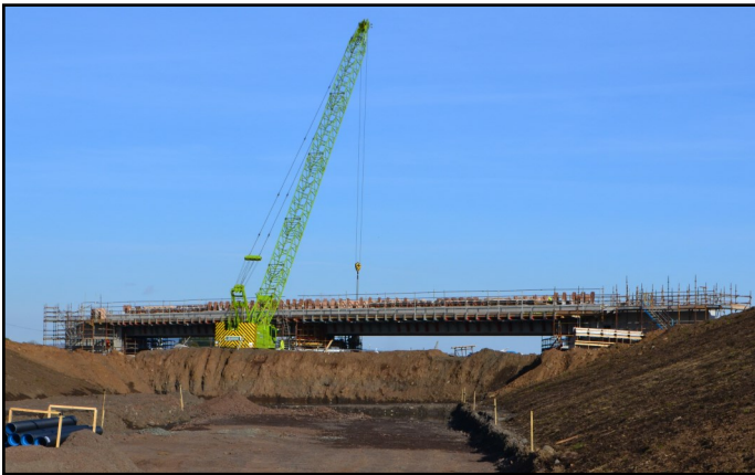
Construction of Derrygowan bridge
