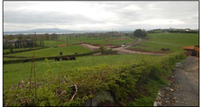
Earthworks commenced on the Randalstown to Toome section of the scheme.
