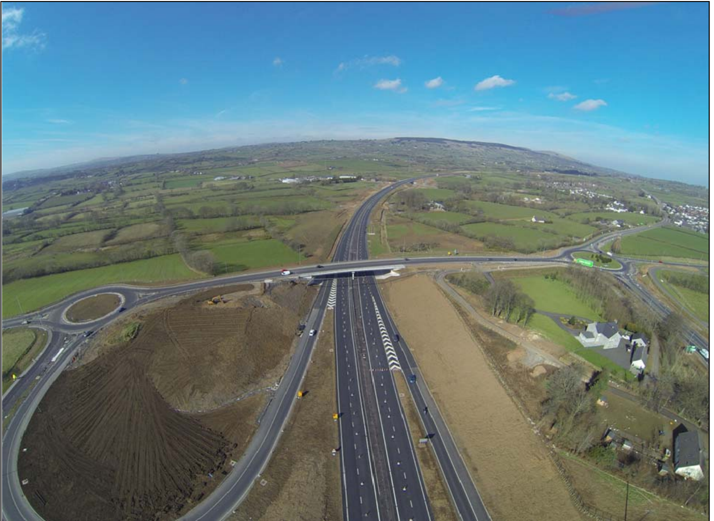
Photograph shows aerial view of the junction connecting the A57 Templepatrick Road to the A8 dual carriageway.
