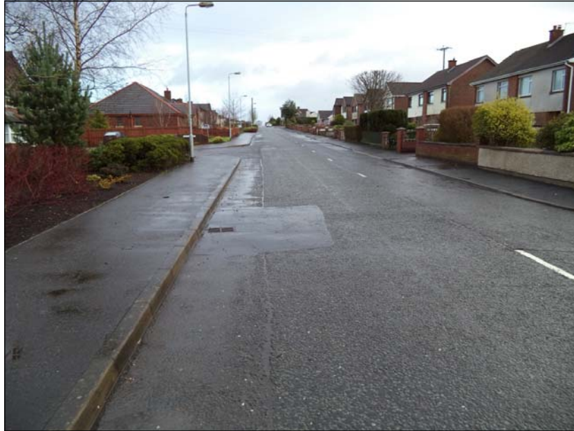
Victoria Road, Traffic Calming (BEFORE)
