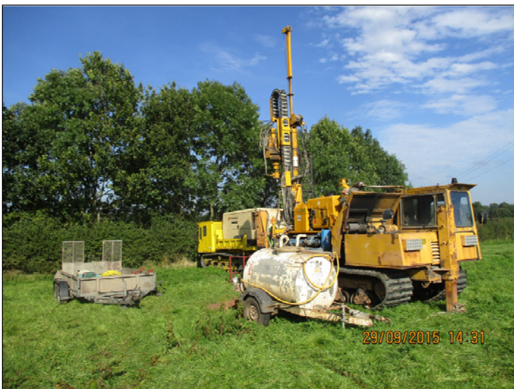
Ground investigation works
