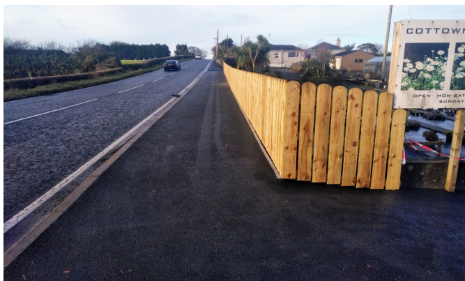
Footway provision completed Nov 2018
