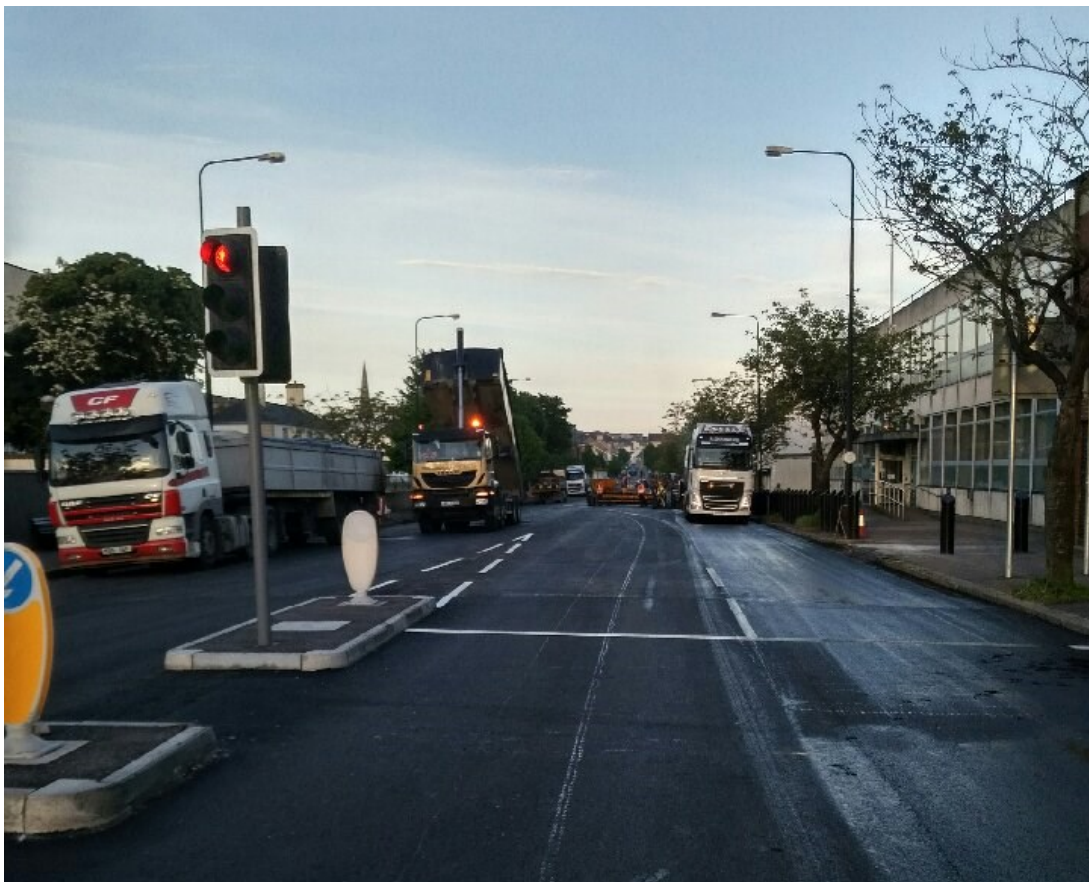
Regent Street , Newtownards Resurfacing and Traffic Signal upgrade
