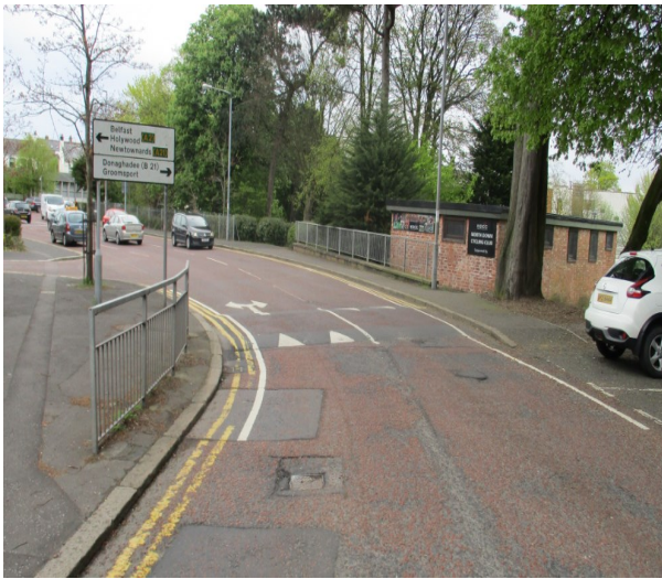
Provision of vertical deflection measures (road humps)
