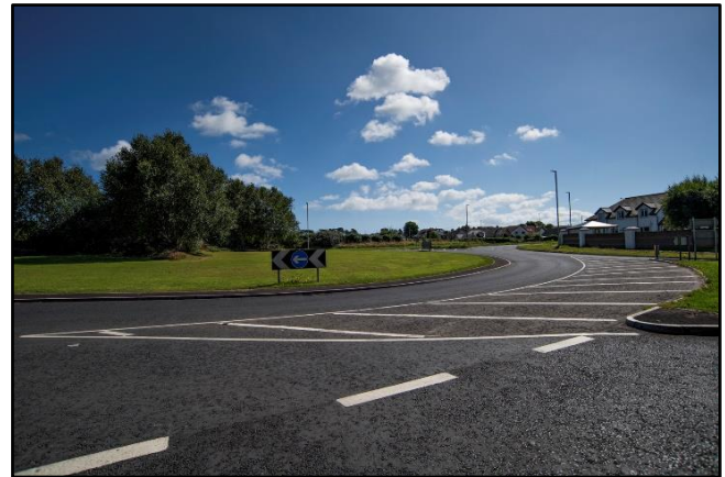
Groomsport Road Roundabout, Groomsport
