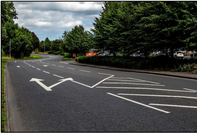
Airport Road West, Holywood
