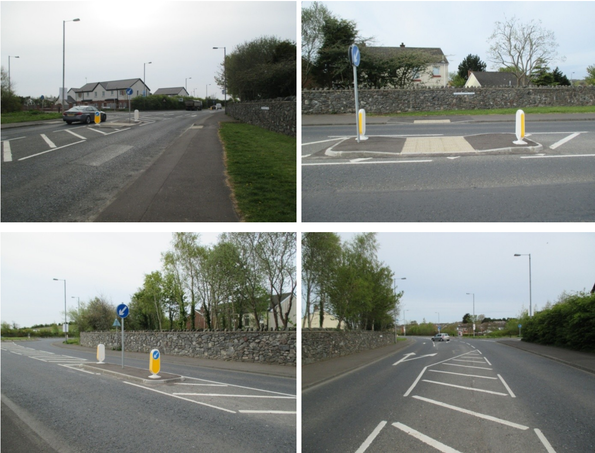
New traffic islands on Newtownards Road, Comber
