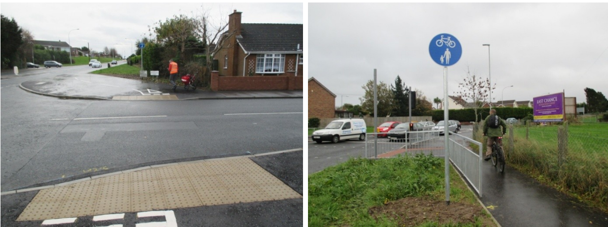
Shared Cycle / Footway facilities on Gransha Road
