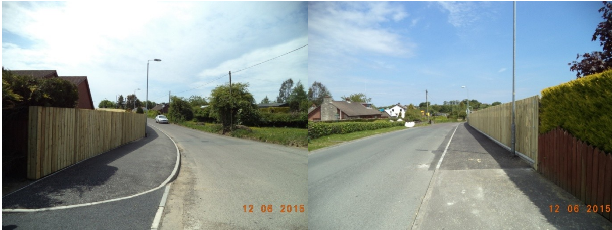
Magherascouse Road—new footway provision
