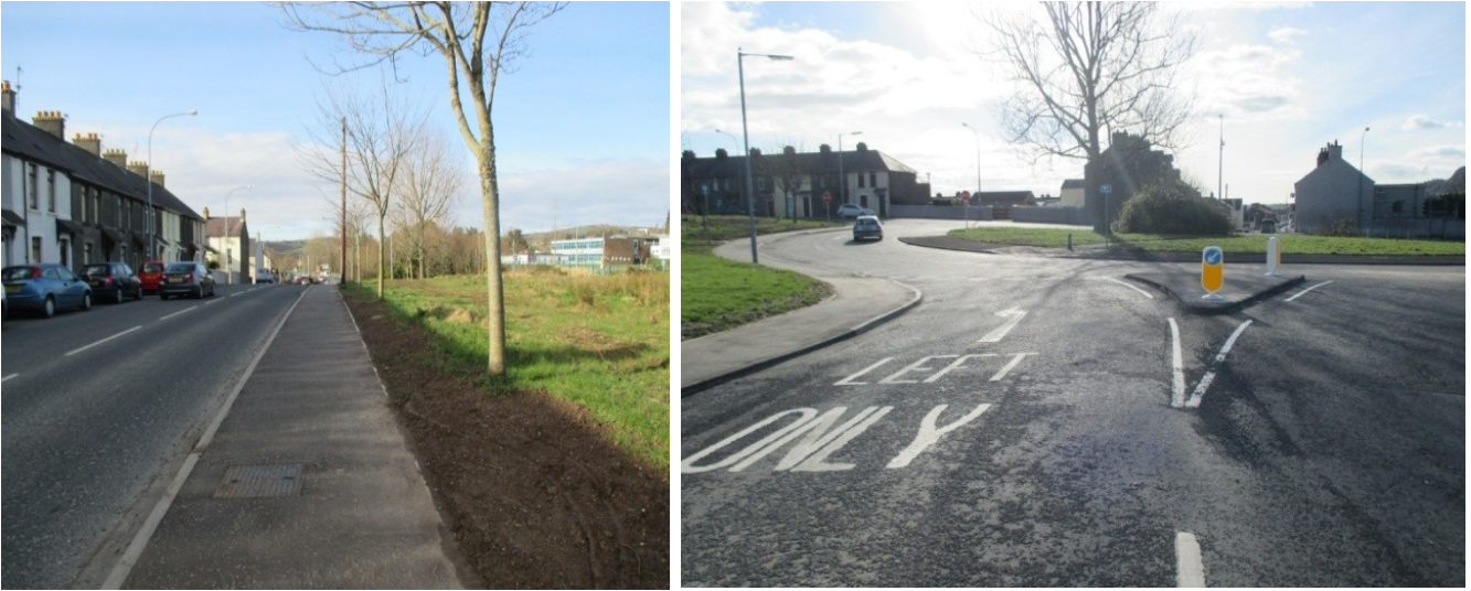
Photographs showing completed infill footway scheme at Talbot Street.
