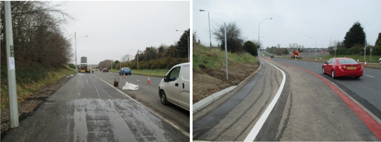
Photographs during construction of new segregated cycletrack / pedestrian footway
