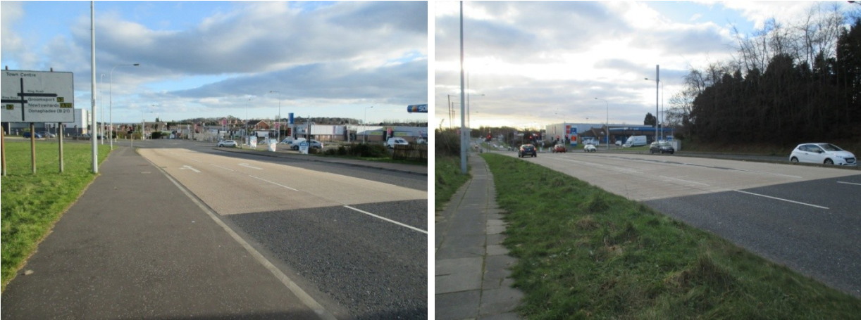
High friction surfacing at the A2 West Circular Road / Clandeboye junction.
