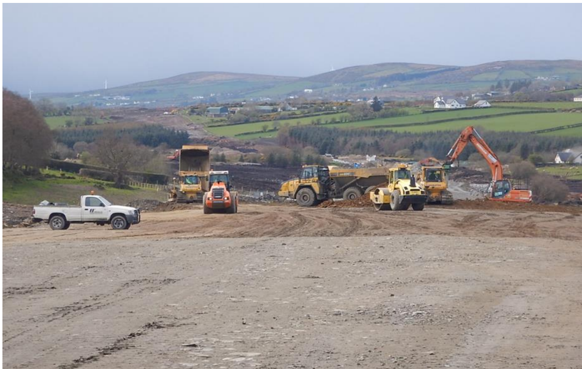
Photo: Construction works at Foreglen
