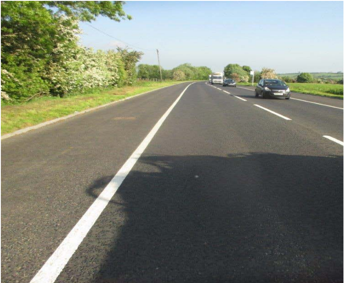
Mulvin Road, Victoria Bridge
