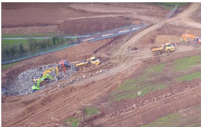
Earthworks commenced on the Randalstown to Toome section of the scheme.
