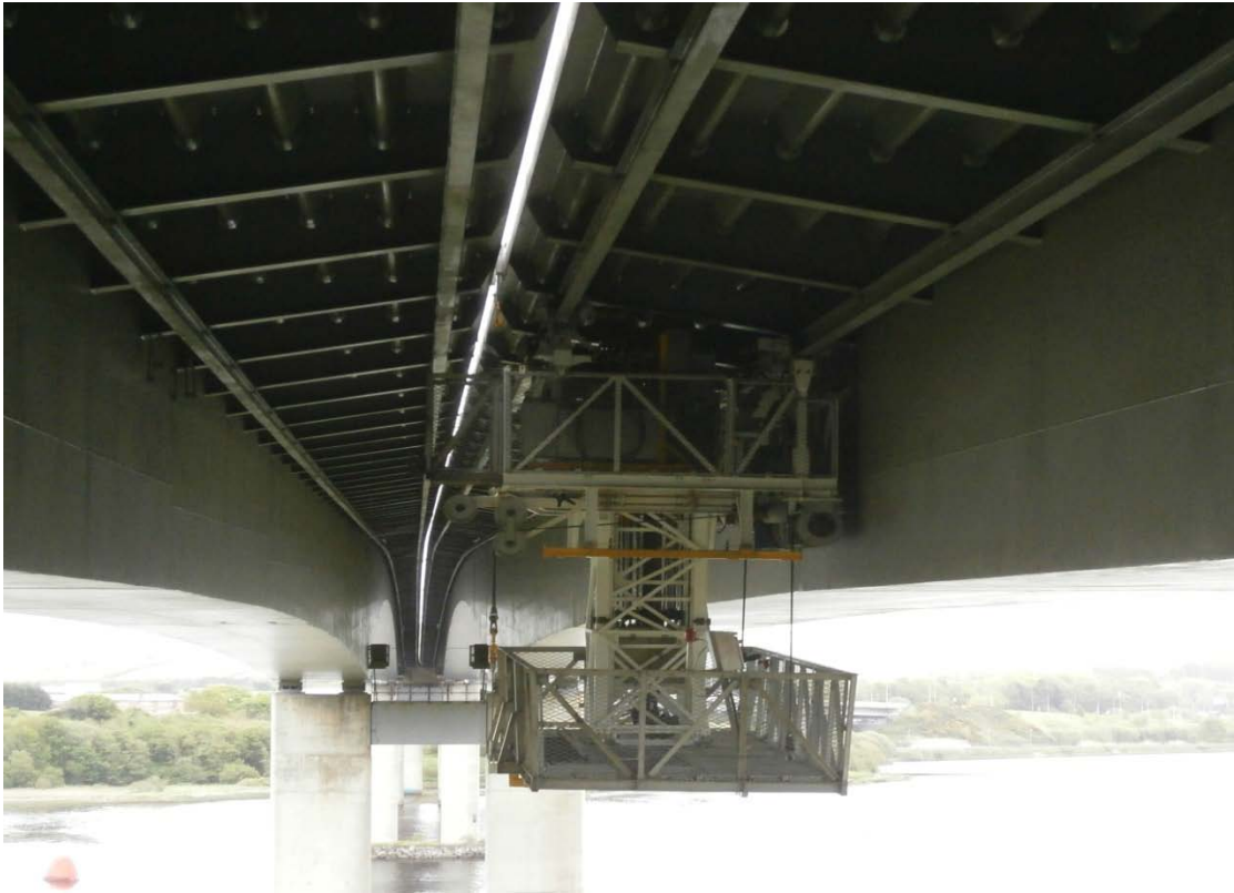
Foyle Bridge - Completion of Gantry Refurbishment
