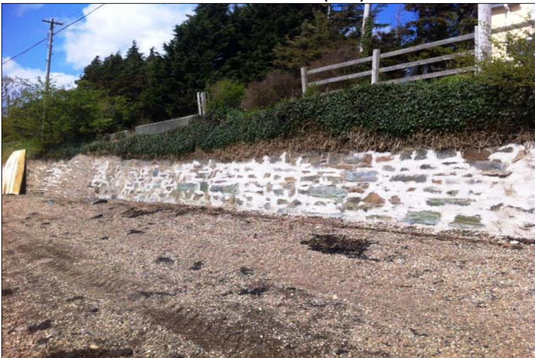
Culmore Point Road (after)
