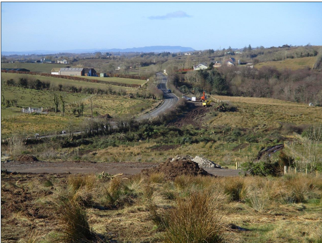
Site Clearance at A32 Cornamuck
