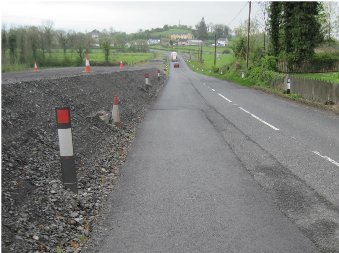
A509 Derrylin Road at Derryhowlaght – Additional ground Surcharge
