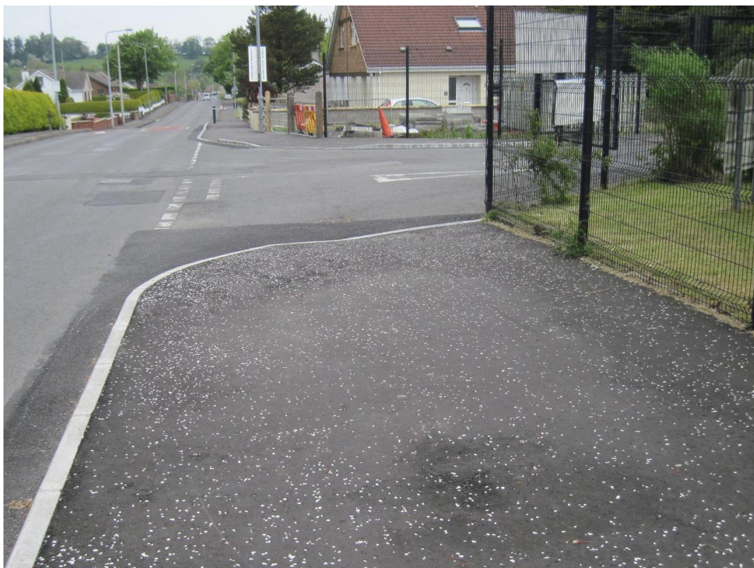
C409 Crevenish Road, Kesh – provision of new set down area and footway link
