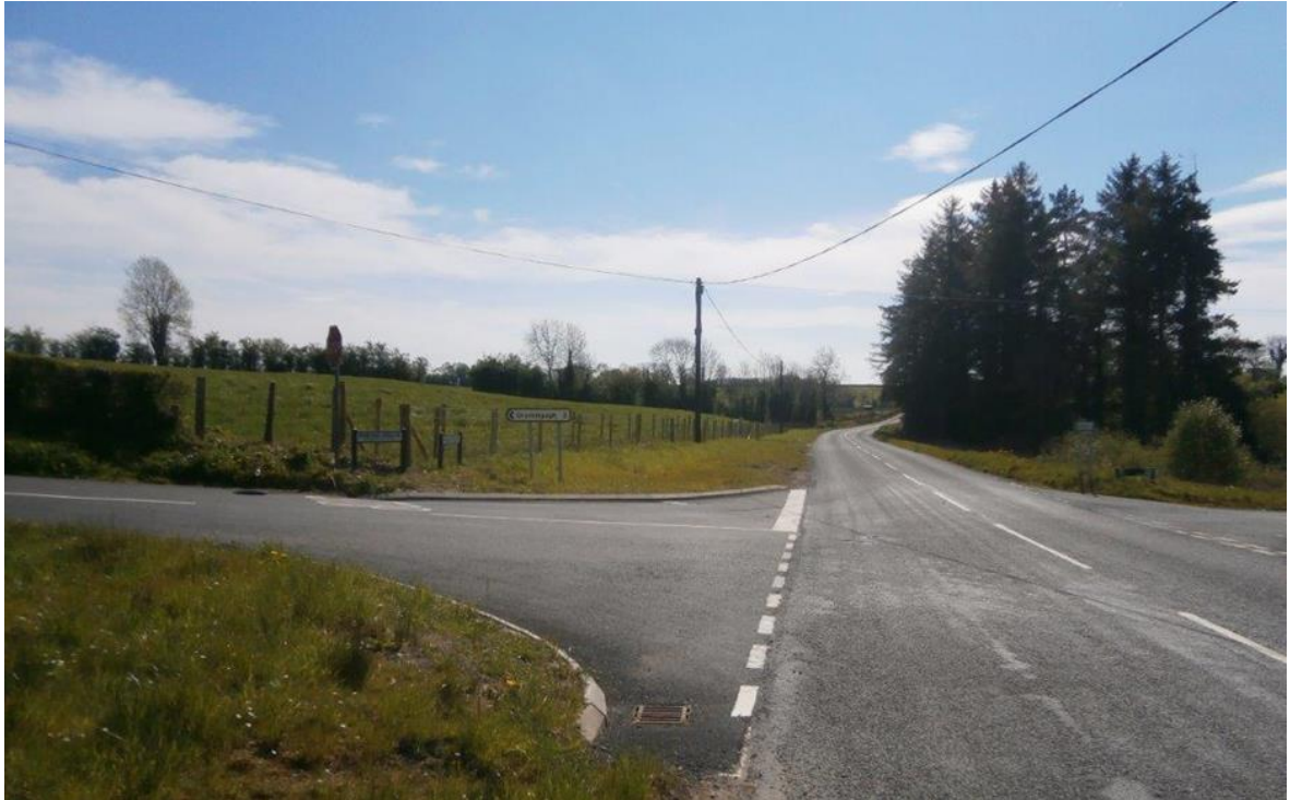
B50/C680 Castleberg Road/Drumlegagh Road – junction sightline improvement
