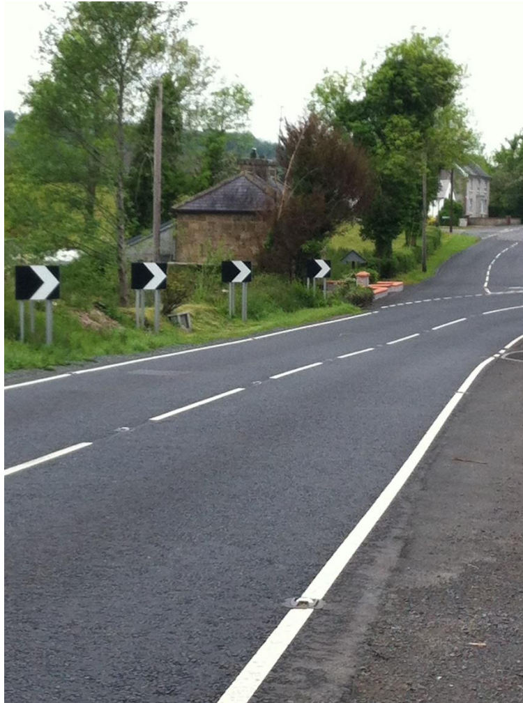
A509 Derrylin Road at “Fatt’s Cross” – provided new chevron boards
