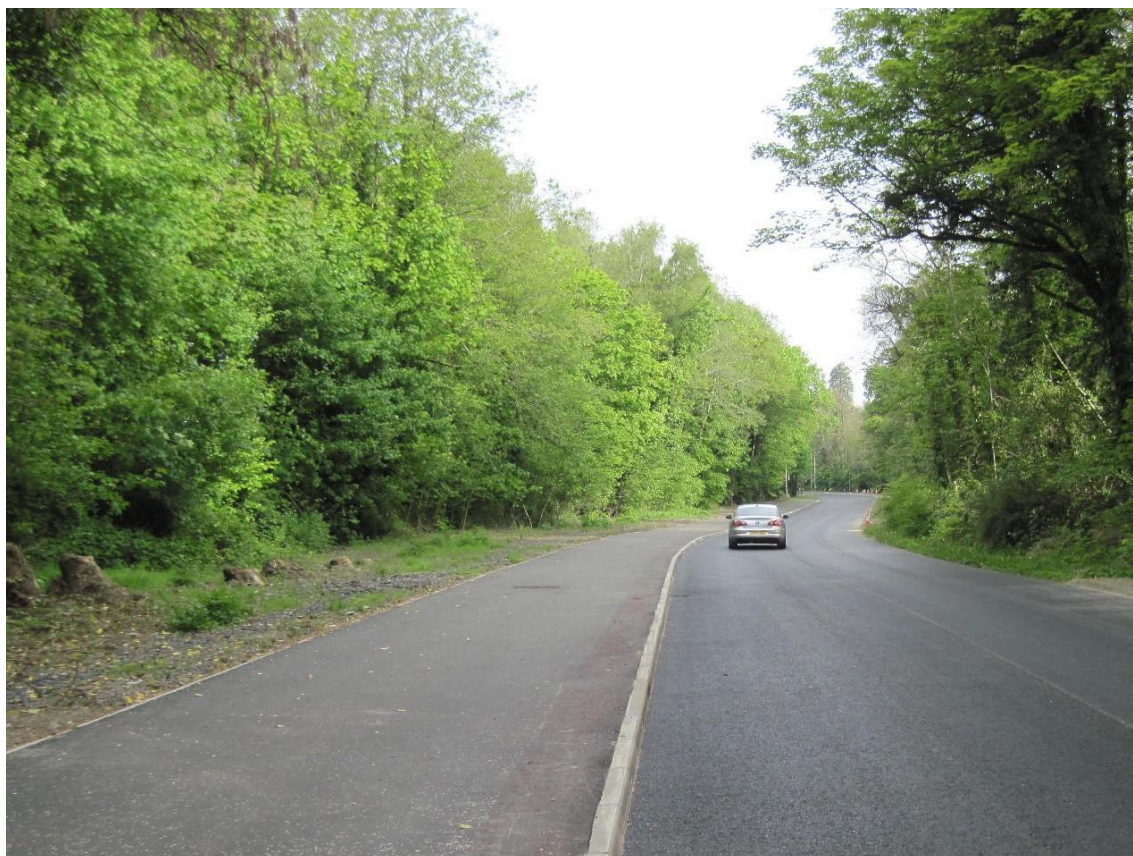
U6513 Lough Yoan Road, Enniskillen – Provided new shared footway/cycleway
