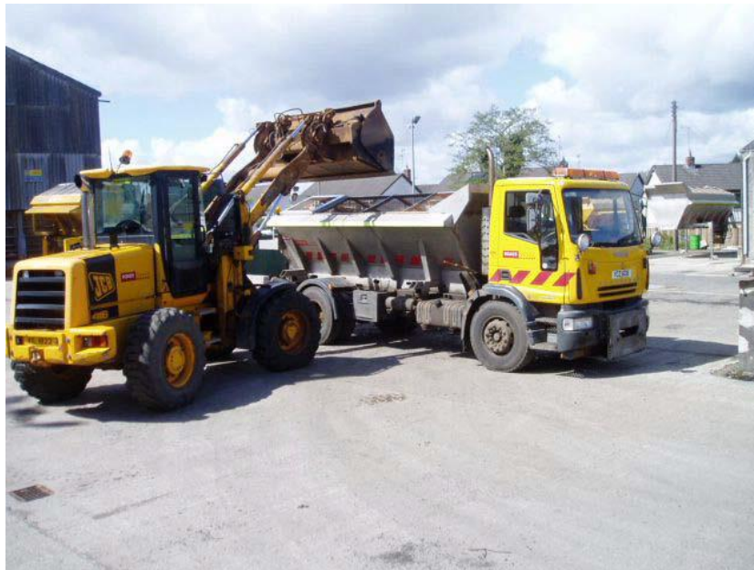
Loading a lorry for a gritting action
