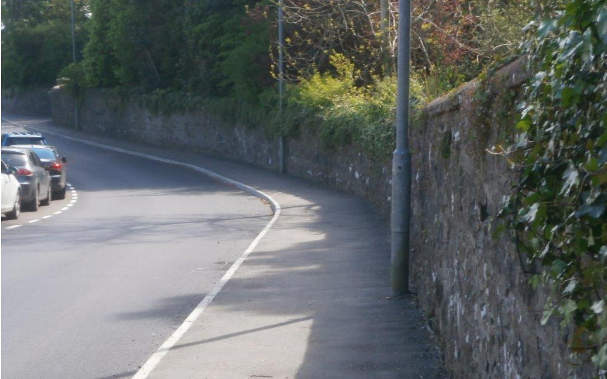
U3005 Brooke Street, Omagh – footway widening
