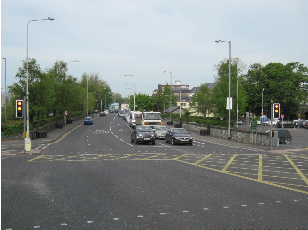
A4 Frith's Pass/Quay Pass, Enniskillen – traffic signals upgrade and junction widening
