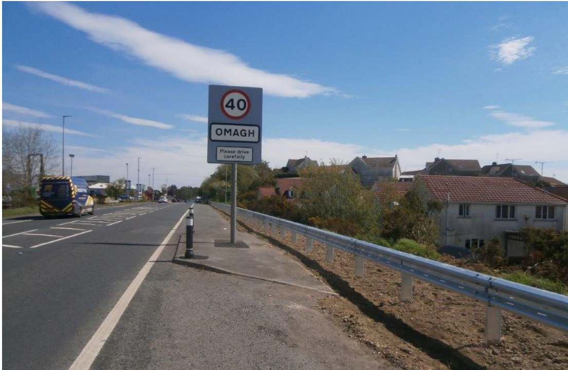
A32 Clanabogan Road, Omagh – Vehicle safety barrier
