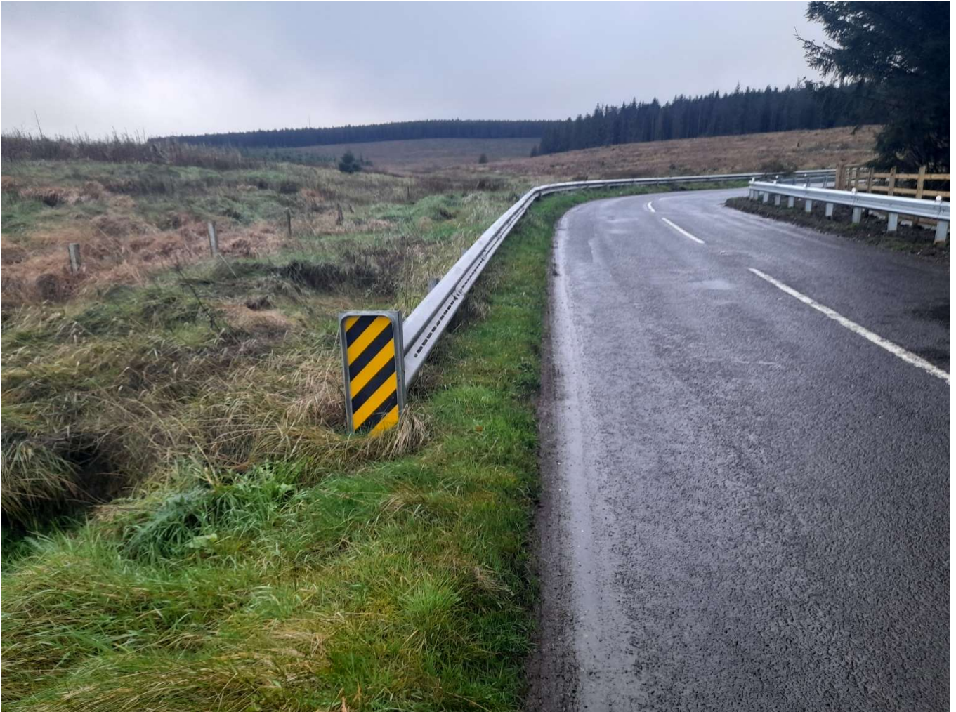
Starbog Road – Upgraded vehicle restraint system.
