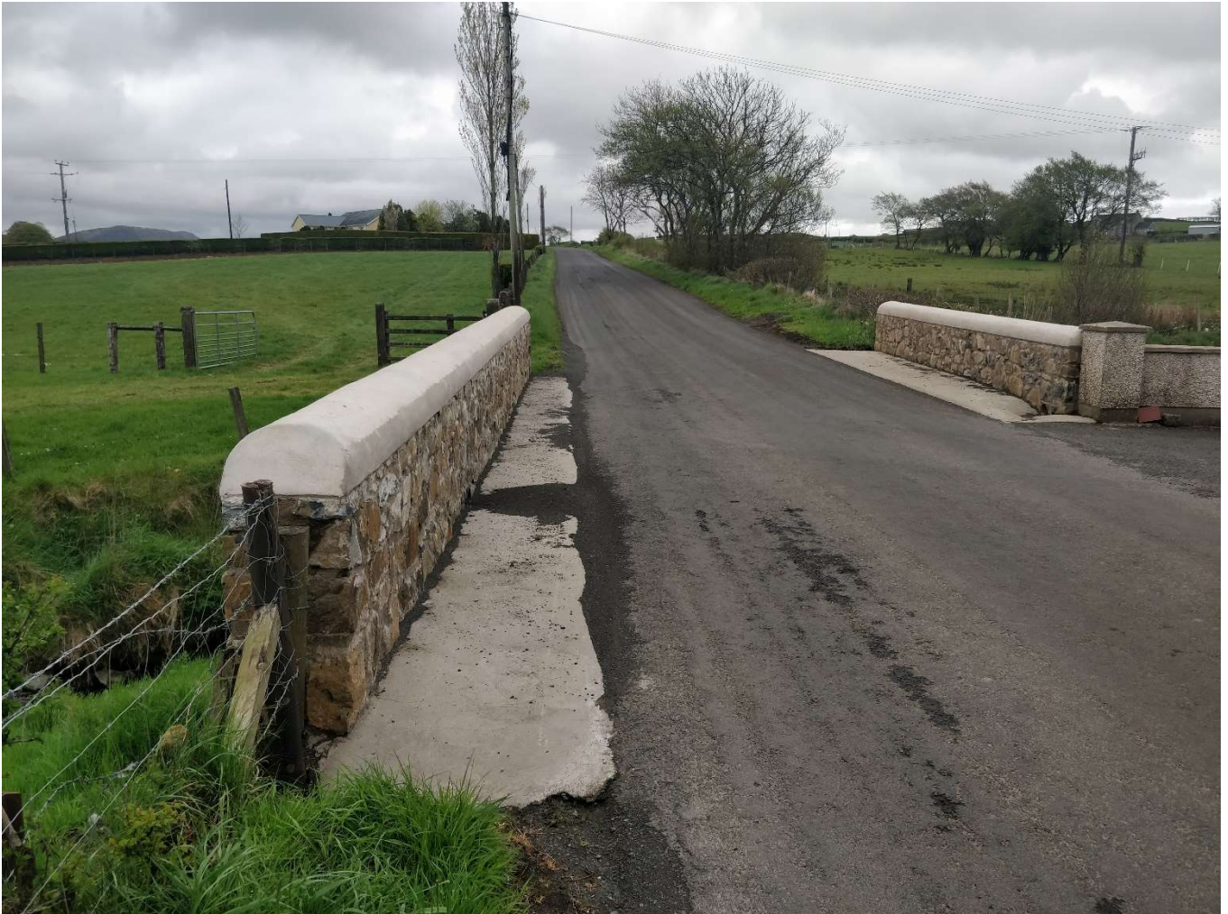
Magillstown Bridge, Lisnahilt Road, Ballymena – Parapet Work
