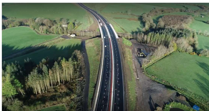
A6 Dual Carriageway over the River Roe.
