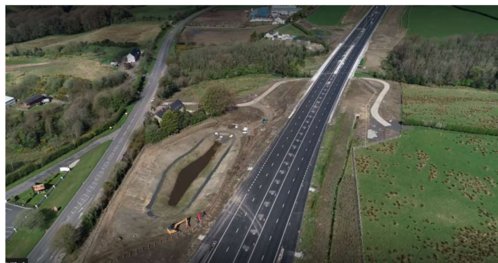
A6 Dual Carriageway at Liberty Glen
