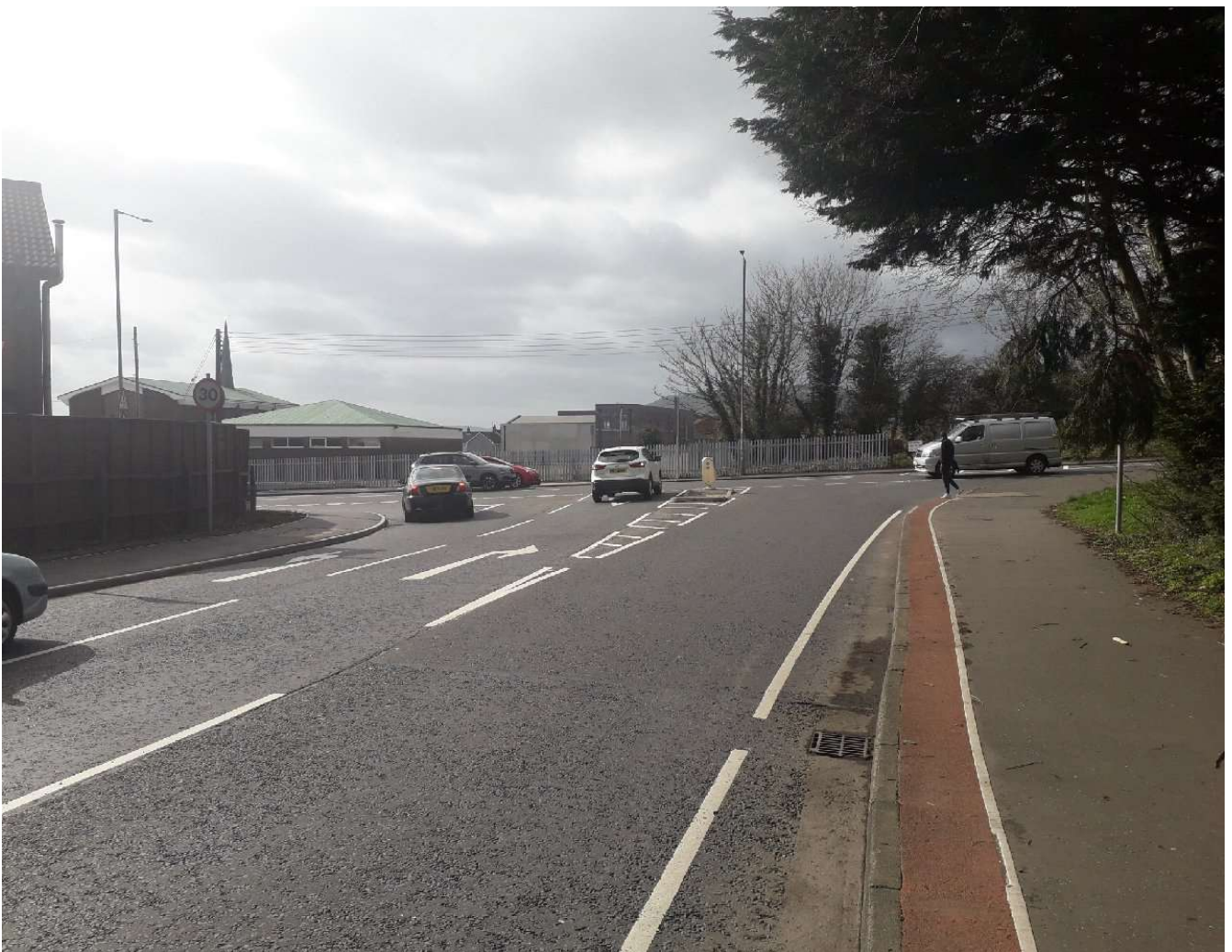
Completed Scheme - Dedicated Left Turn Lane. Prince Andrew Way, Carrickfergus.
