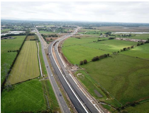
Arial view looking west – Toome Bypass tie-in
