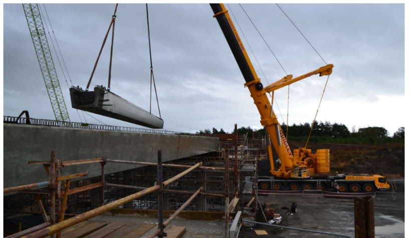
Final beam lift at Hillhead junction overbridge
