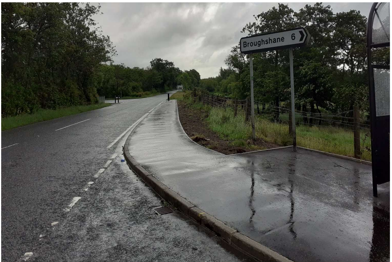
Completed Scheme – Glenravel Road
