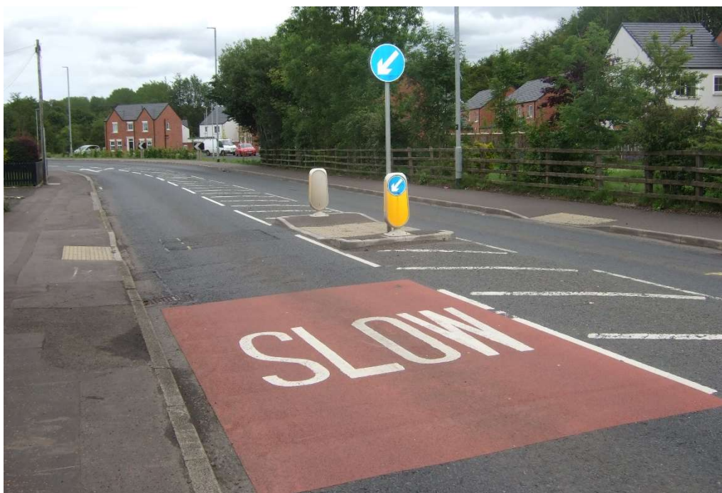
Completed scheme on Fry’s Road, Ballymena
