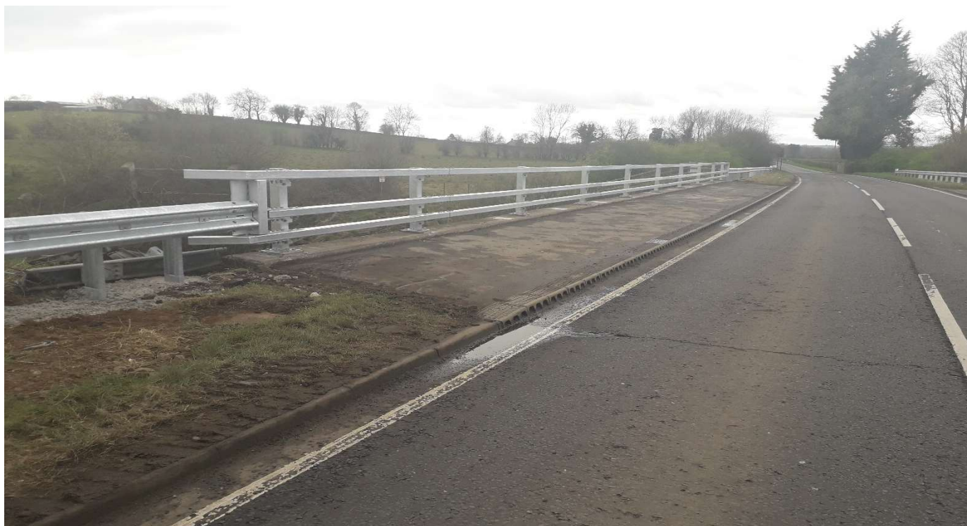
Completed Scheme - Slaght Bridge, Ballymena
