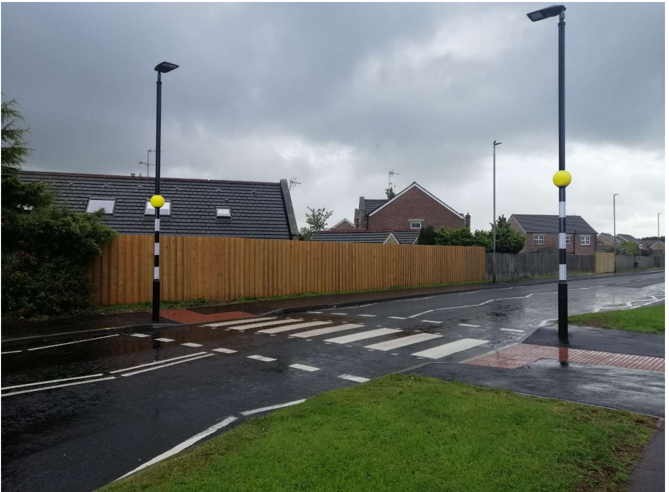
Completed Scheme – Tullygarley Road, Ballymena
