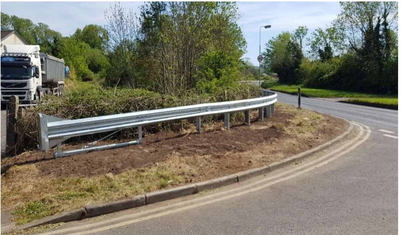
Completed Scheme - Roguary Road, Toome
