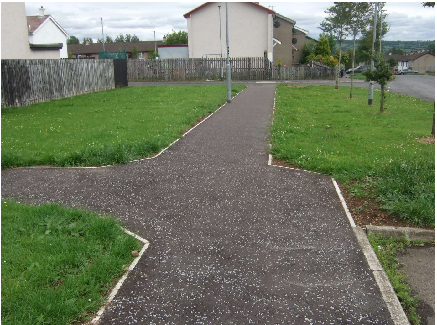
Completed footway scheme at Dunclug Park, Ballymena
