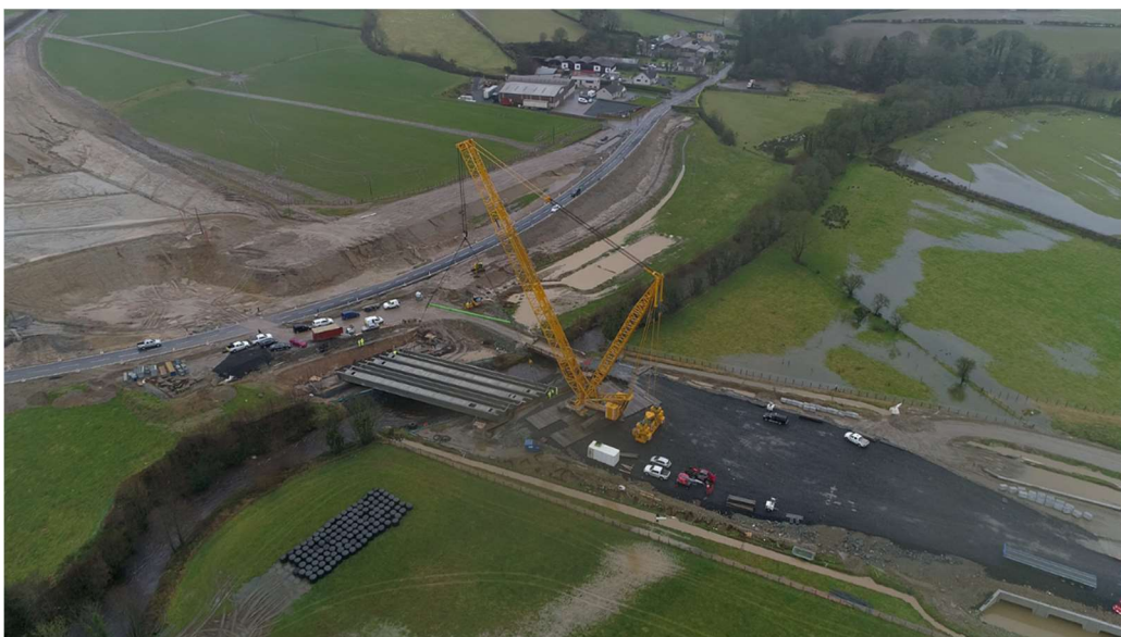
Beams being installed on the Owenrigh River Bridge
