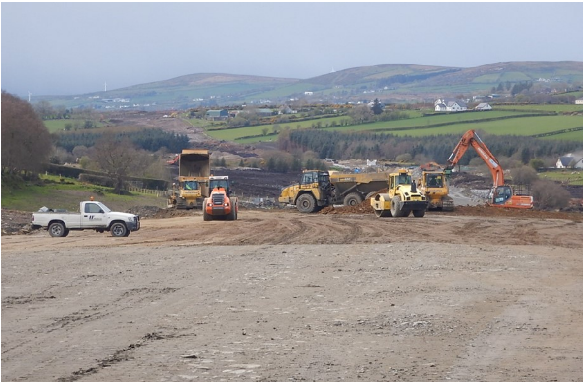
Construction works at Foreglen
