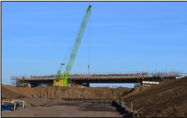
Construction of Derrygowan bridge
