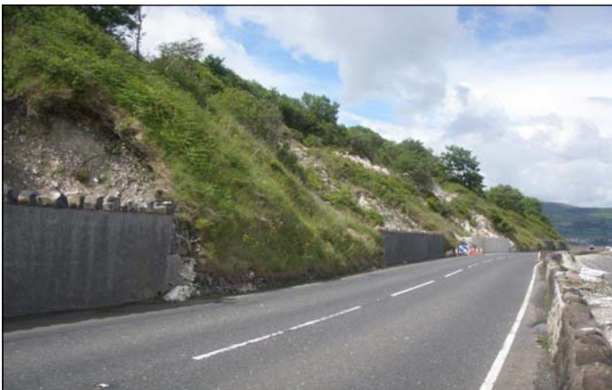
A2 Coast Road, Glenarm - Slope Stabilisation Proposed Scheme - £200,000
