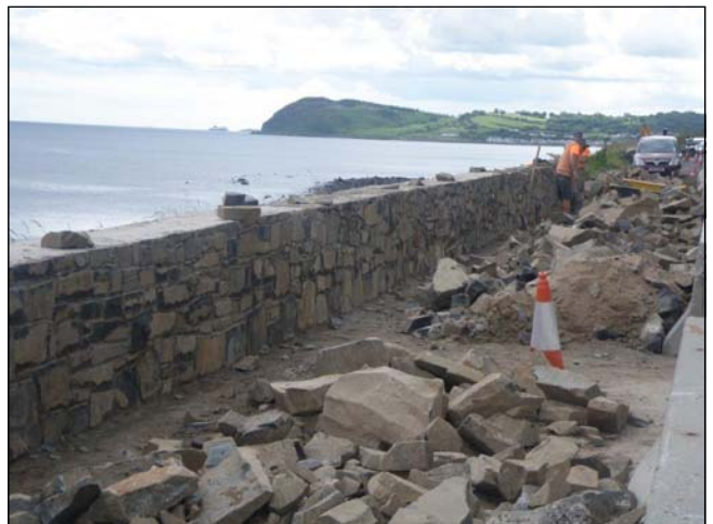
A2 Coast Road, Ballygalley New Parapet Walls - £100,000
