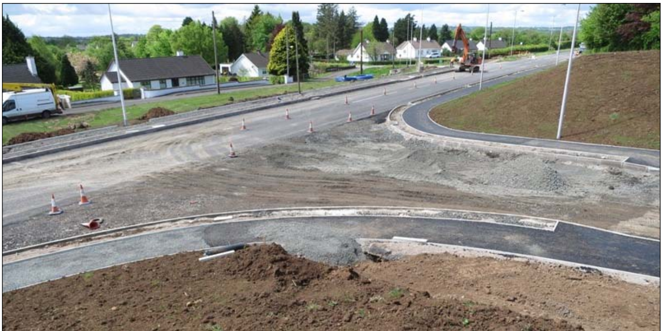
Construction work progressing on site
