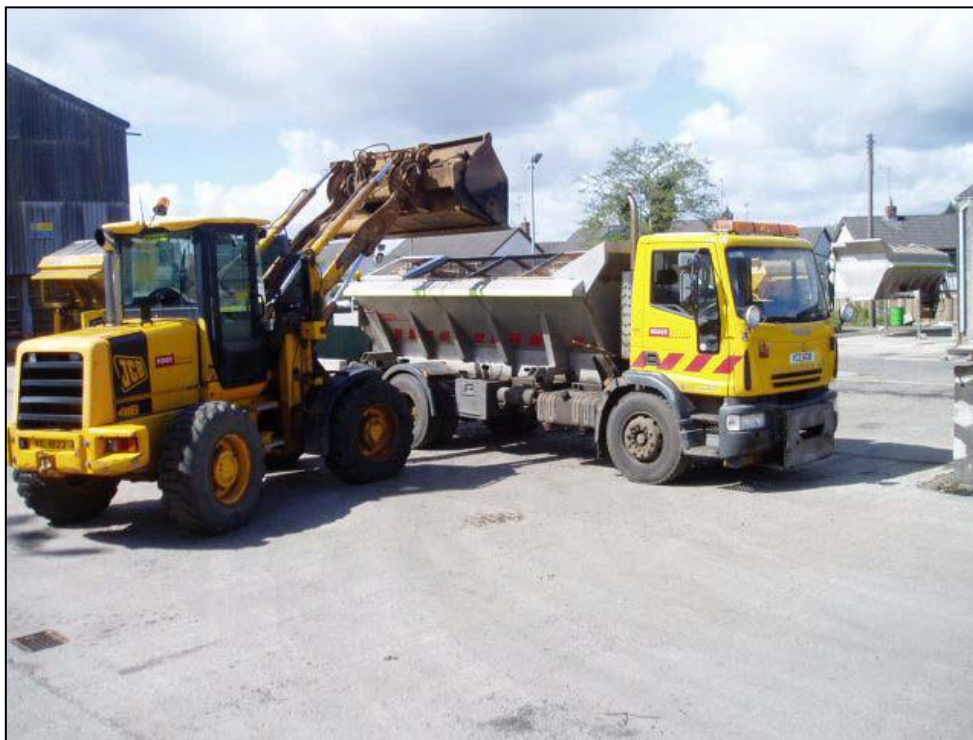
Salt loading one of the gritting lorries
