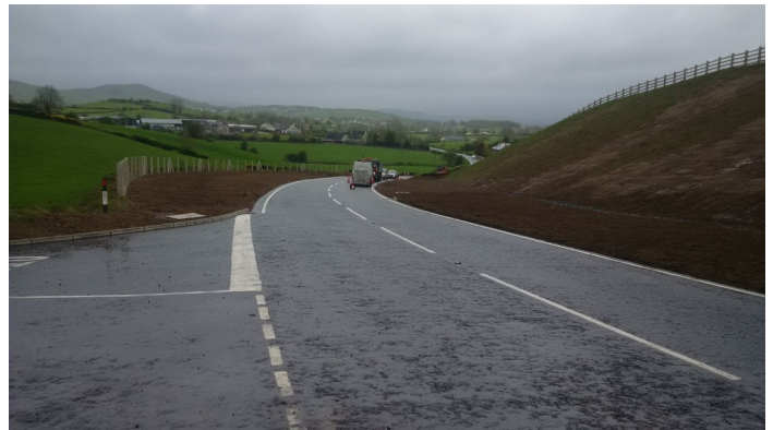
After works were completed on the B8
