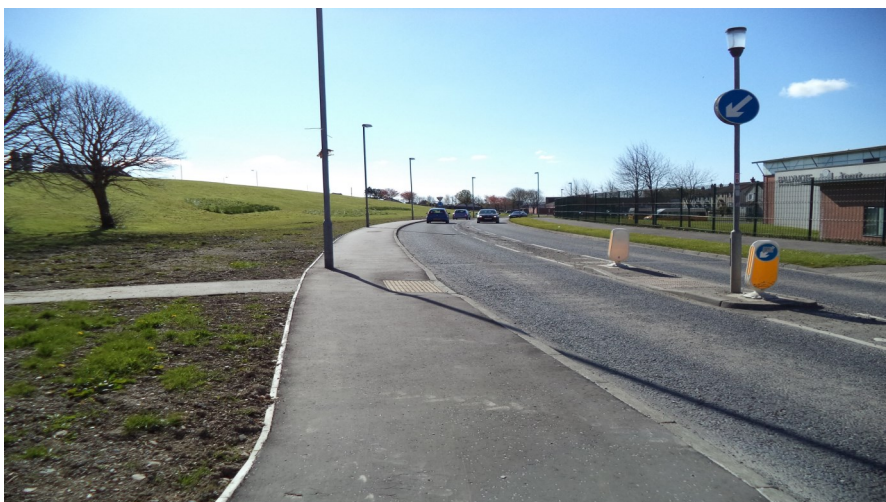
New footway completed
