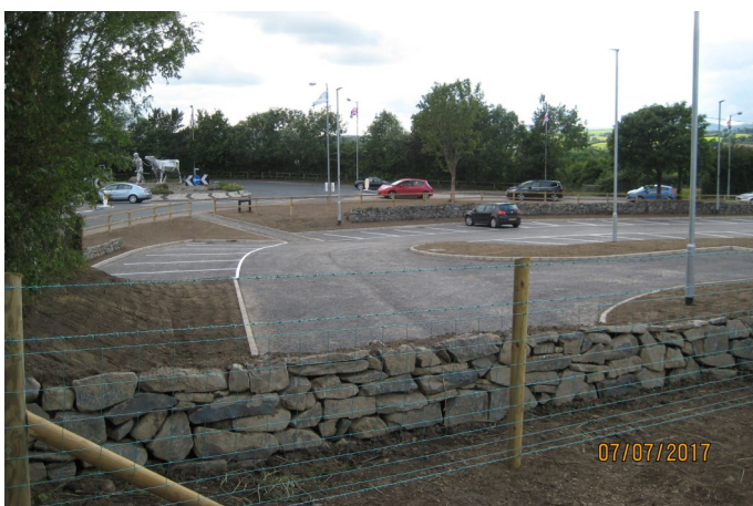
Completed scheme on opening
