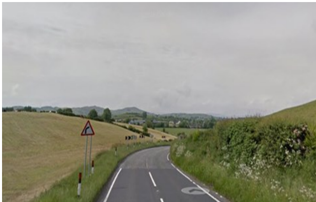
Before B8 road alignment improvements
