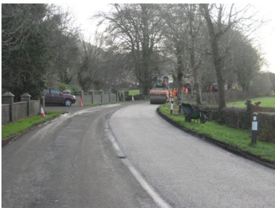
During carriageway resurfacing work
