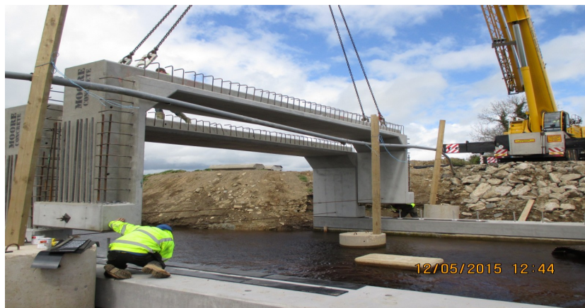
Bridge under construction
