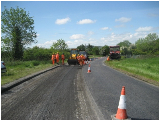
During carriageway resurfacing work
